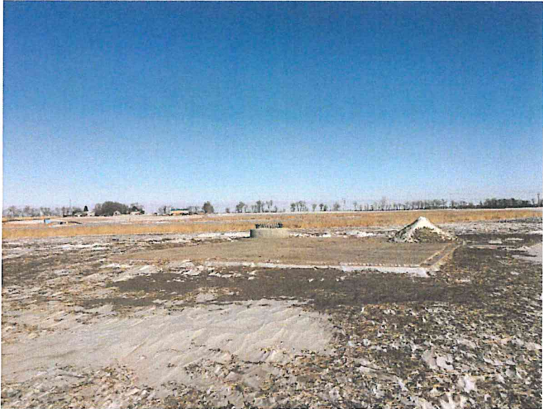
Example of Mats placed around the foundation Foundation No. 6 Looking E.
