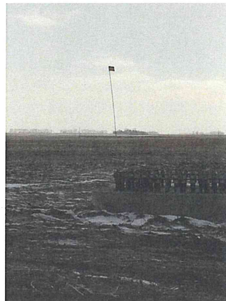
Foundation No. 13 Looking W.
