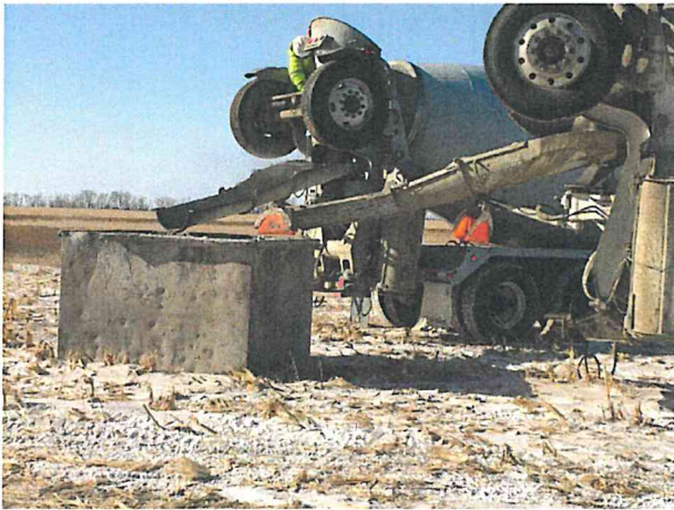
Foundation No. 8 Looking E.
