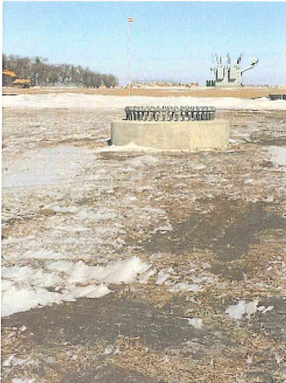
Foundation No. 1 Looking N.
