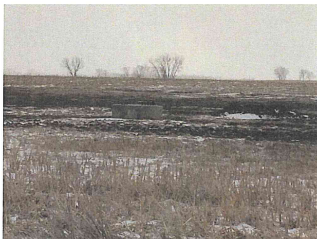
Foundation No. 37 Looking E.
