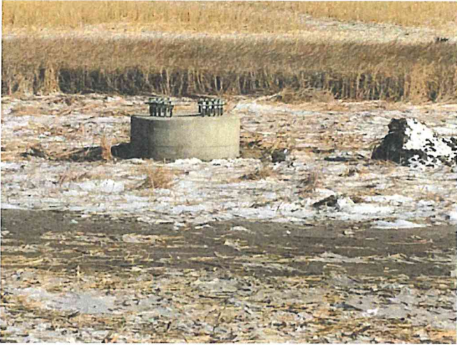
Foundation No. 5 Looking S.
