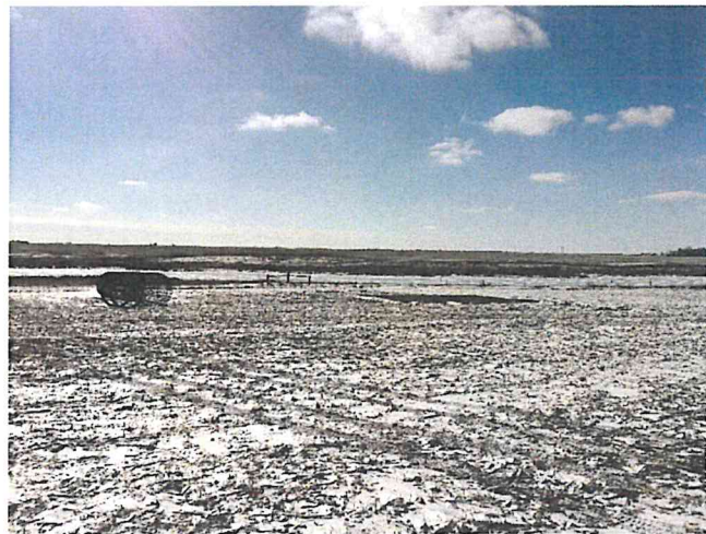
Foundation No. 15 Looking S.
