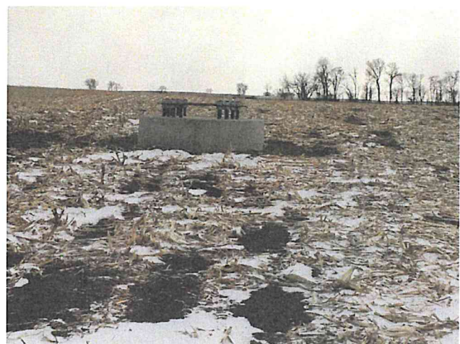
Foundation No. 38 Looking E.
