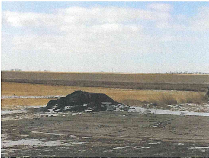
Foundation No. 18 Looking E.
