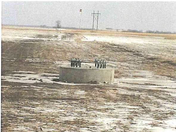
Foundation No. 29 Looking E.
