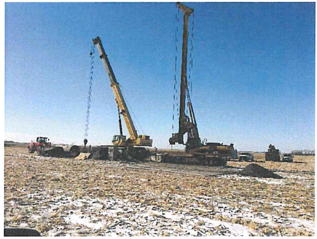
Foundation No. 11 Looking SW.
