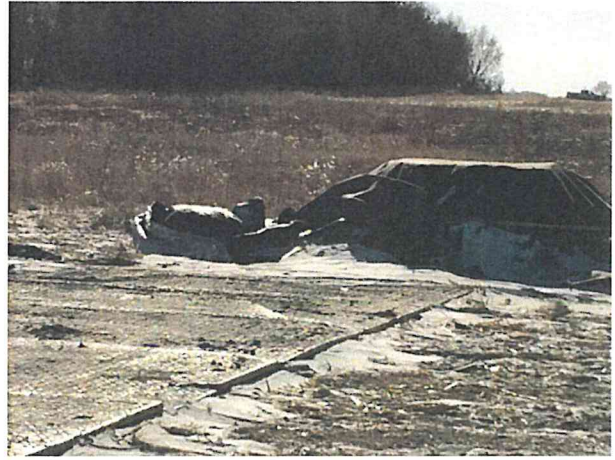
Foundation No. 9 Looking S.
