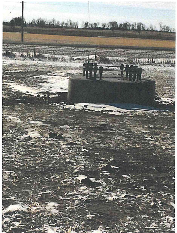
Foundation No. 2 Looking S.
