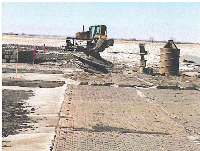
Foundation No. 12 Looking W.
