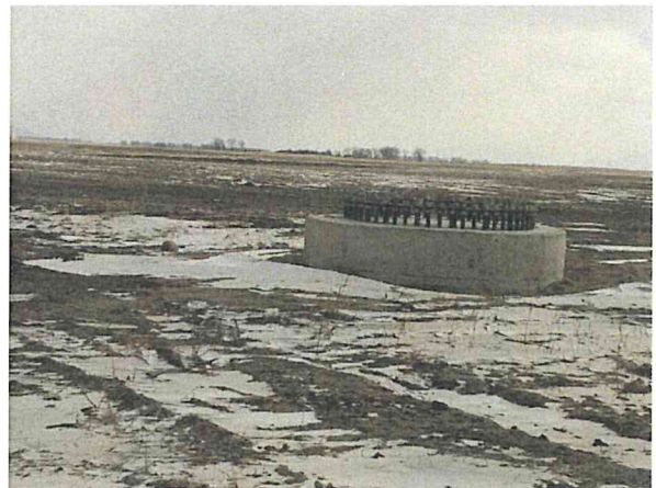
Foundation No. 30 Looking S.
