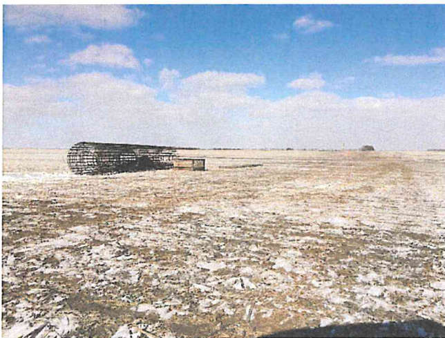
Foundation No. 14 Looking SW.
