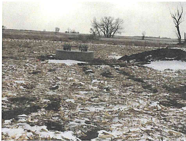
Foundation No. 39 Looking E.
