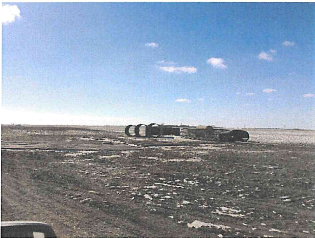
Foundation No. 10 Looking SW.
