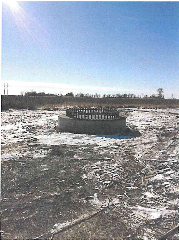
Foundation No. 3 Looking W.
