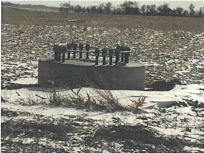
Foundation No. 16 Looking W.
