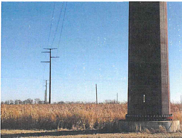
Base of Pole No. 003 Looking SE
