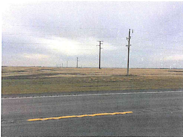
Power Poles 019, 018, 017 Hwy. 281 Looking W.
