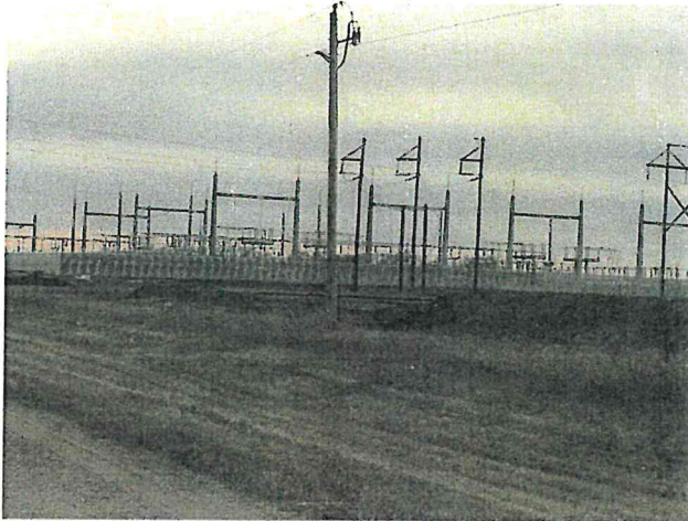
Completed Ellendale Substation Looking SE
