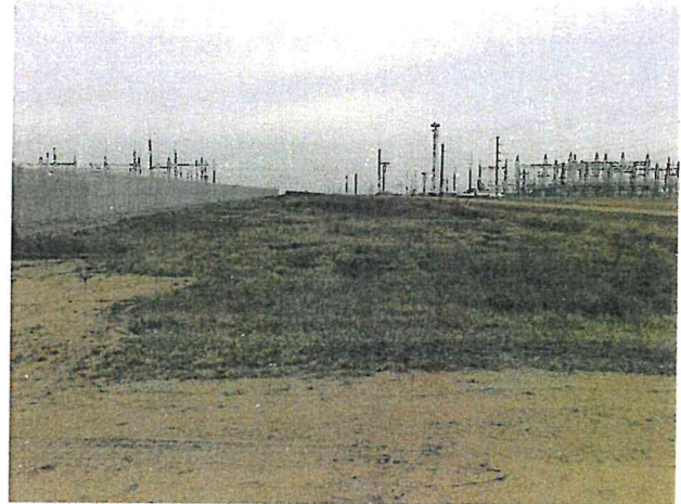
Completed Road Right of Way on East Side of Substation Looking North
