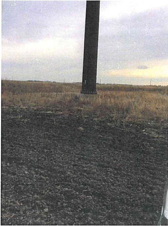
Base of Power Pole No. 007 Looking W
