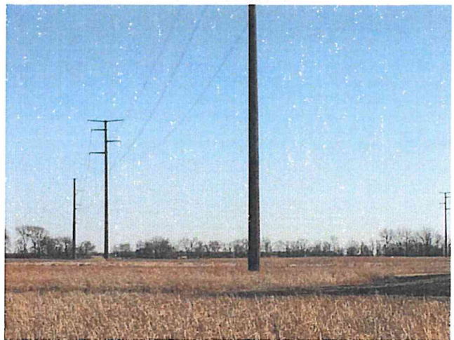
Power Poles 004, 005, 006 Looking East
