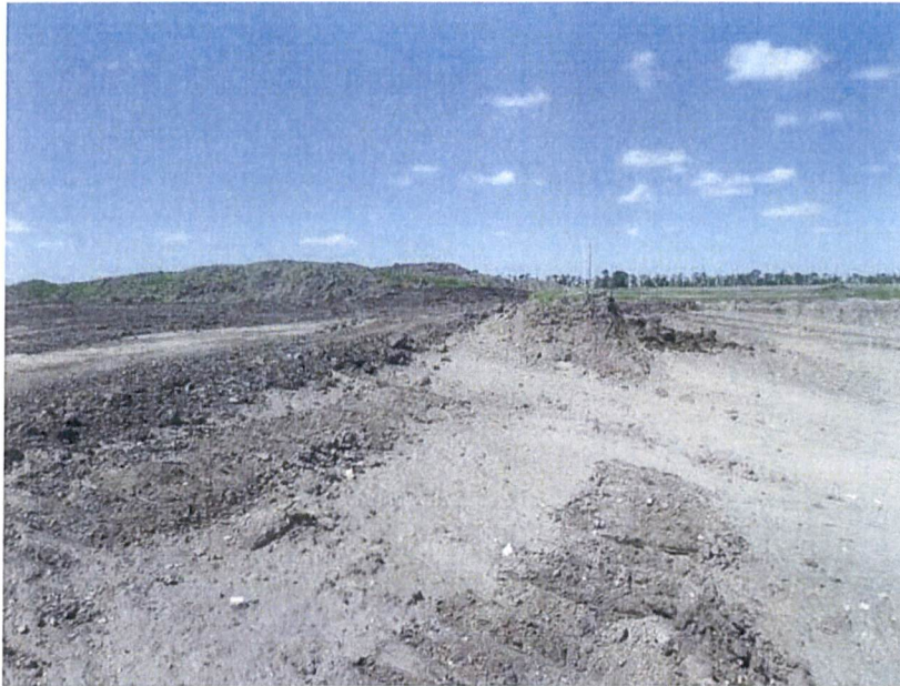
Photo 5: Pedestal showing topsoil depth. Subsoil removal occurring to right of the pedestal and topsoil removal occurring left of the pedestal. In the background is a ridge of topsoil that has been pushed up with a dozer and is waiting to be removed by shovel and truck.
