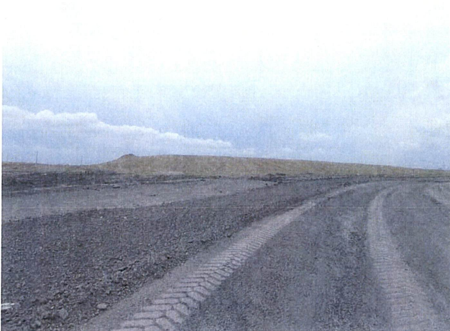
Photo 4: This pile is composed of the overburden mentioned in Photo 3. It is to be used as a subsoil replacement in Ash Pit 118 (Sec 3).
