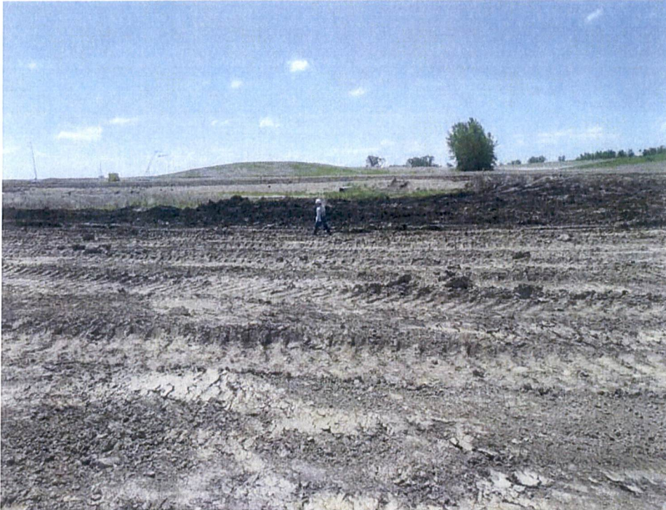
Photo 7: Photo shows an area of sodic topsoil. This topsoil is chemically unsuitable for use as SPGM and has been cut out of the lift area.
