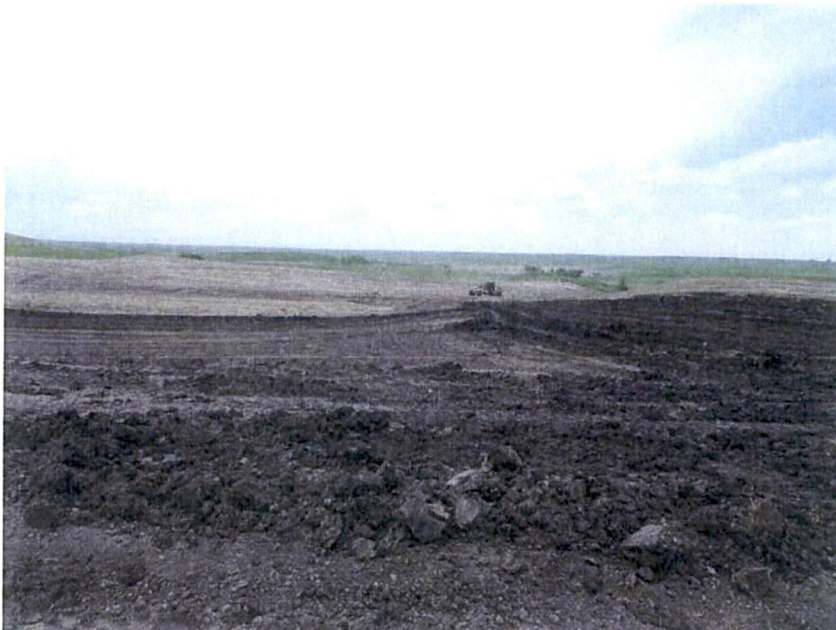
Photo 2: Actively re-spreading topsoil from Photo 1 at the “Butterfly Pit”.
