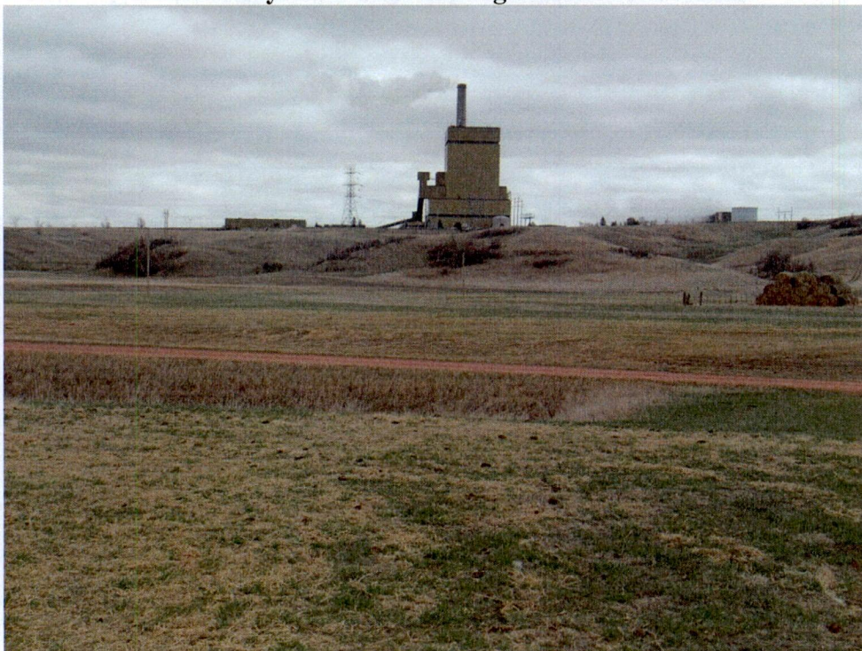
View of Coyote Station looking south across Site 1
