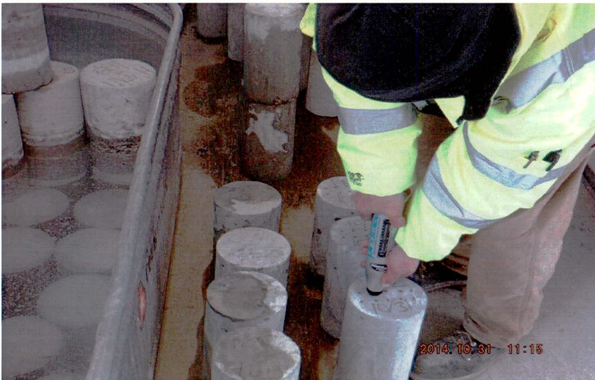
Border Winds – Schmidt Hammer Testing T49 Cylinders
