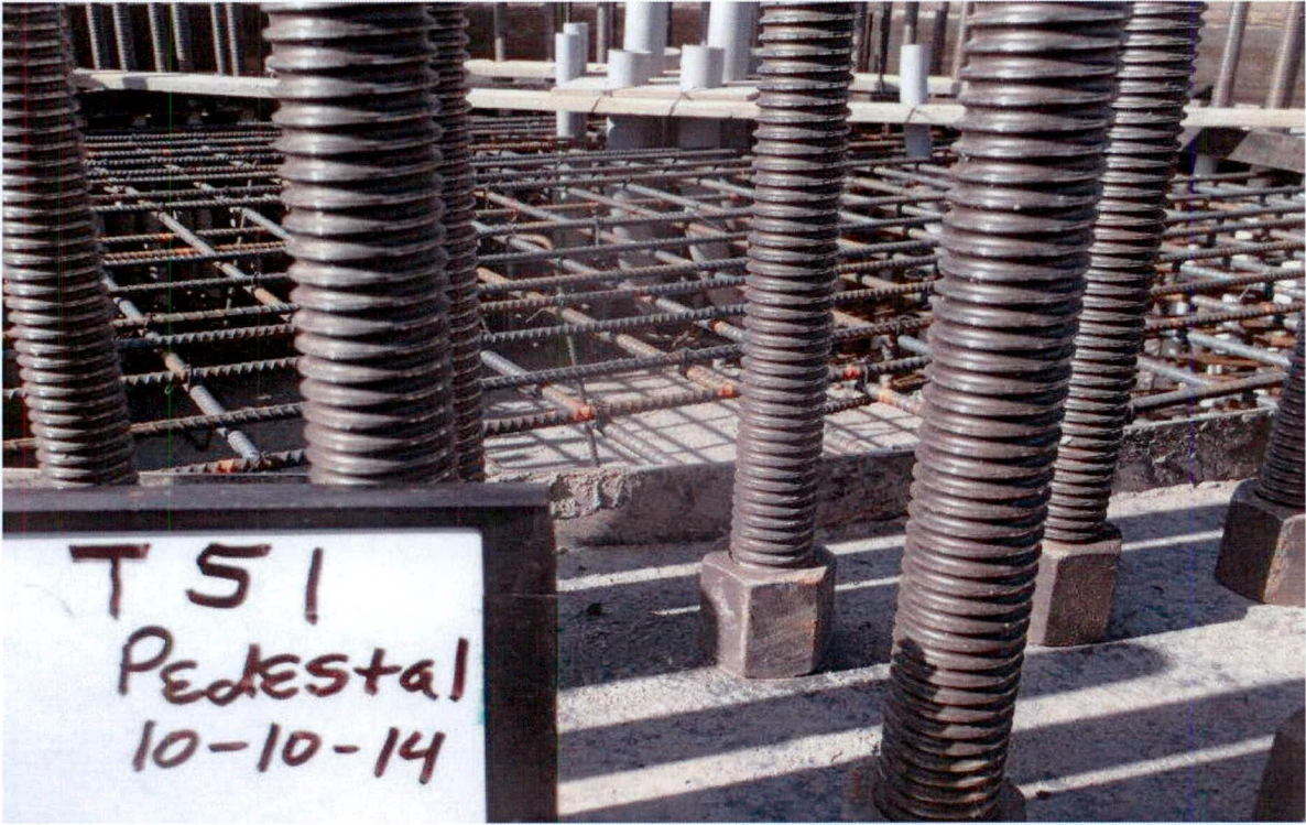
Border Winds; T51 Rebar and conduit
