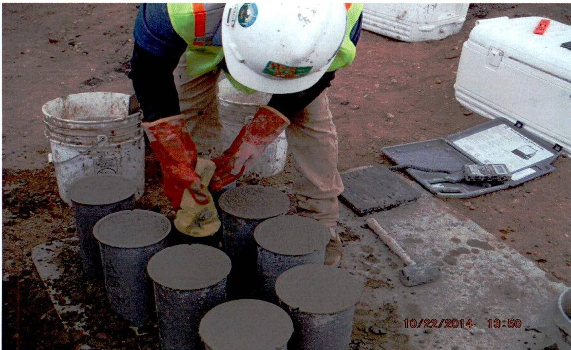
Border Winds - T19 Foundation Concrete Sampling
