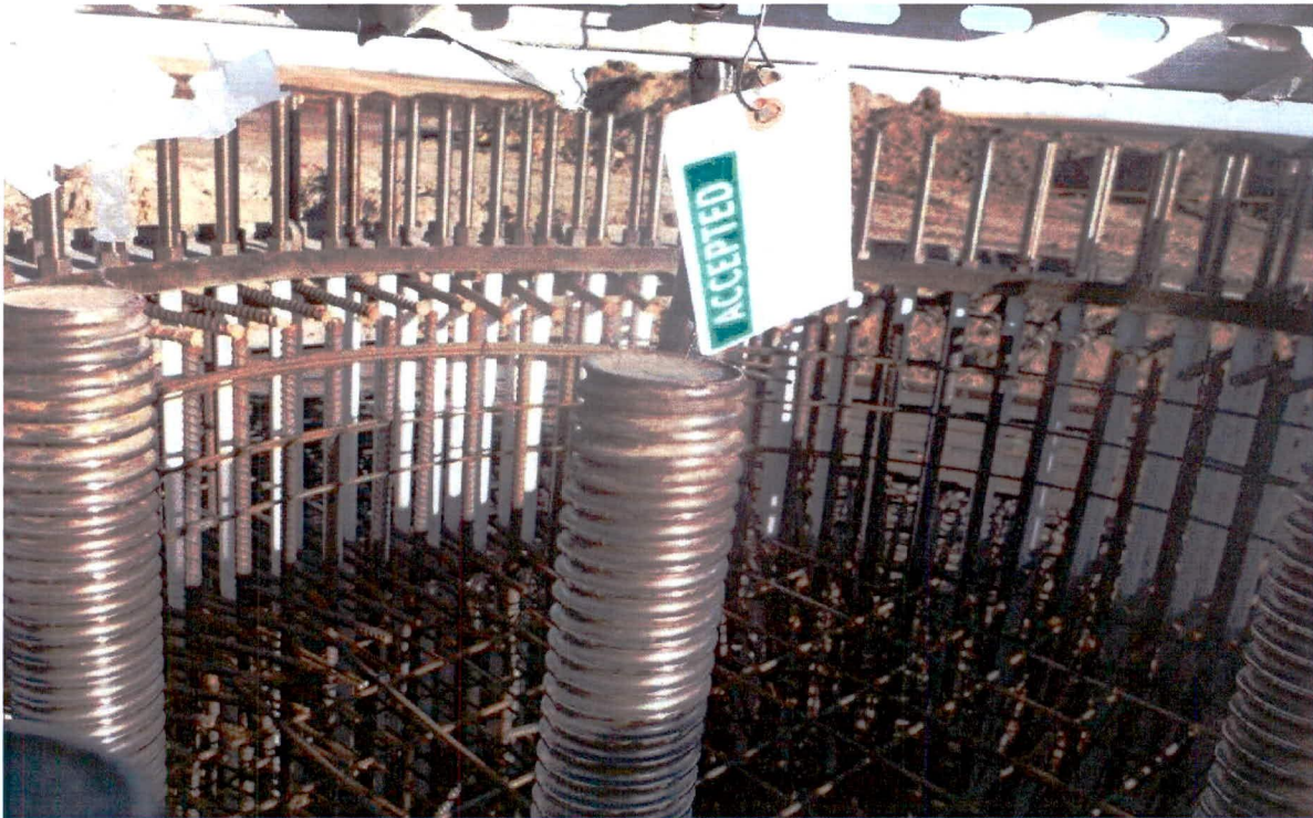
Border Winds; T21 Foundation rebar inspection approval tag
