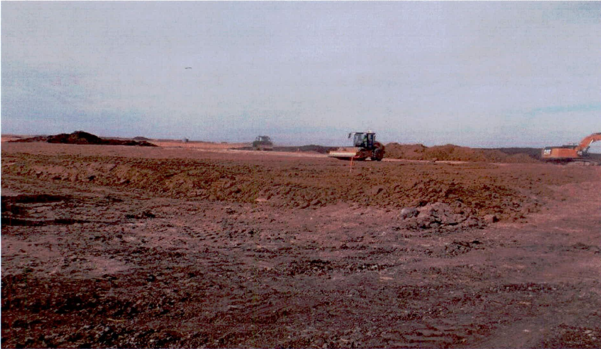
Border Winds; Substation site grading
