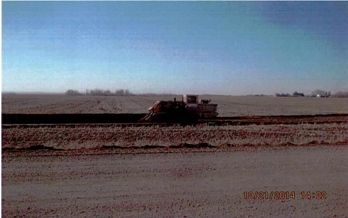
Border Winds - Trenching Operations
