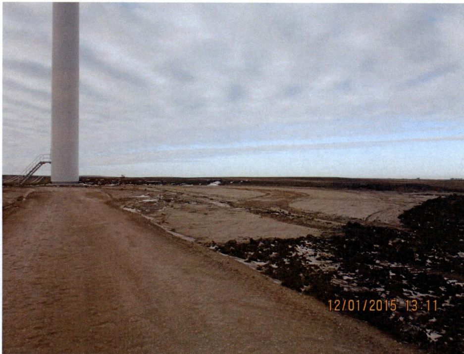
Figure 4. Turbine pad to be reclaimed at T20.
