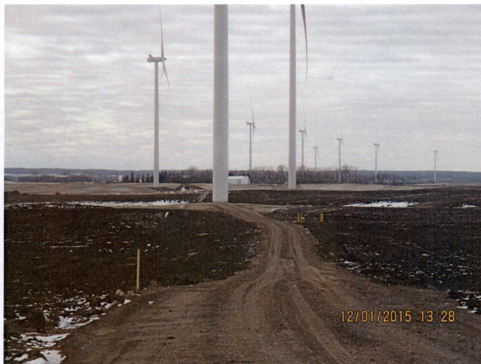
Figure 5. Photo of a service road to be realigned to be in line with the turbine pad at land owner's request.
