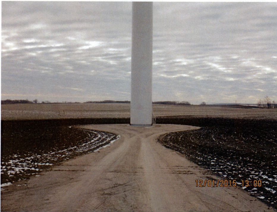
Figure 3. Finished turbine T19 and pad. Topsoil has been disked and service road has a slight taper away from turbine base.
