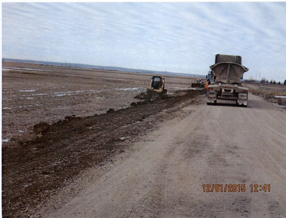
Figure 2. Topsoil being moved back into place and rocks being separated.
