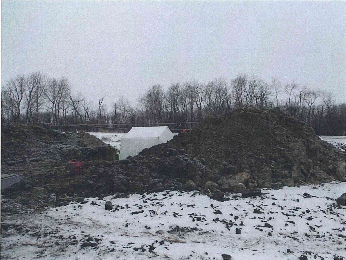
Border Winds – Splice Pit Tent
