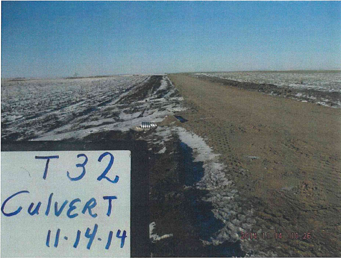
Border Winds – T32 Culvert Installation
