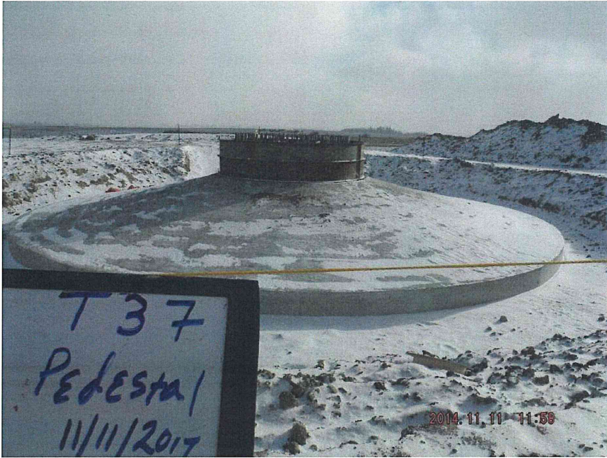
Border Winds – T37 Foundation Pedestal Formed for Pour
