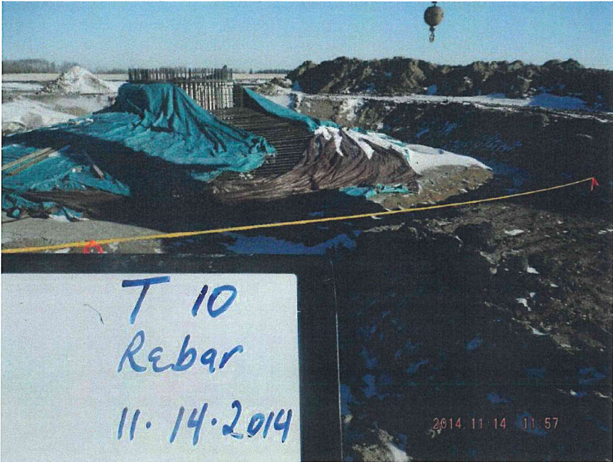
Border Winds - T10 Foundation Rebar Placed
