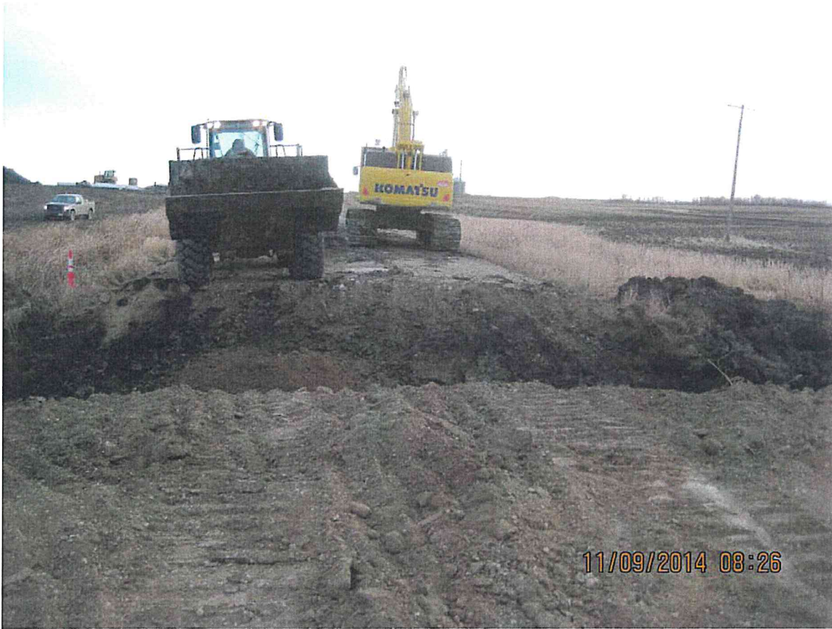
Border Winds – Culvert Installation on 106 th Street
