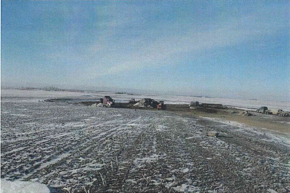
Border Winds: Foundation Backfill
