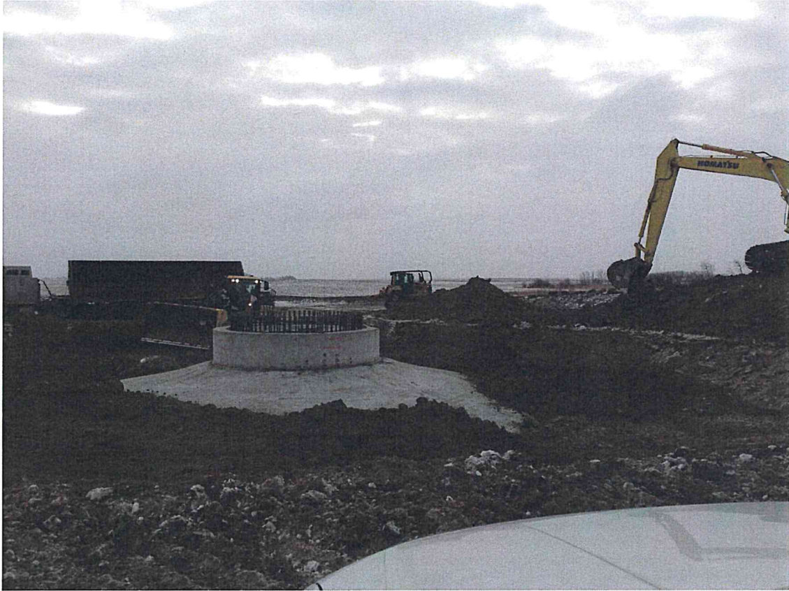
Border Winds: Foundation Backfill
