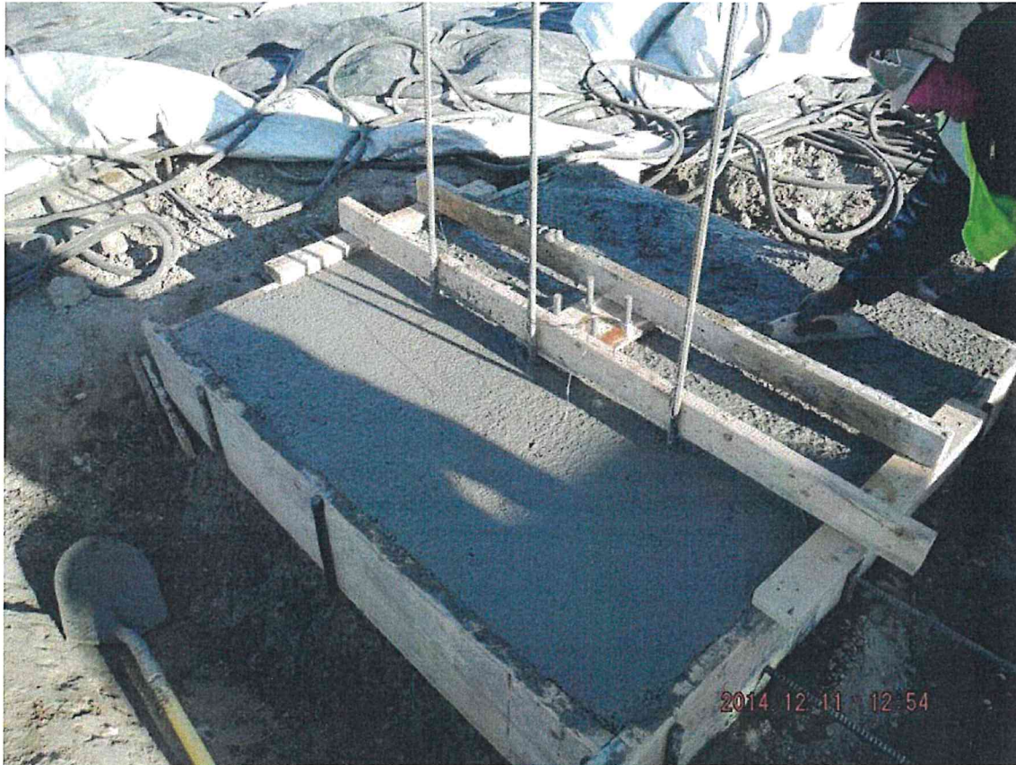
Border Wiinds: O&M Building Interior Foundation Poured
