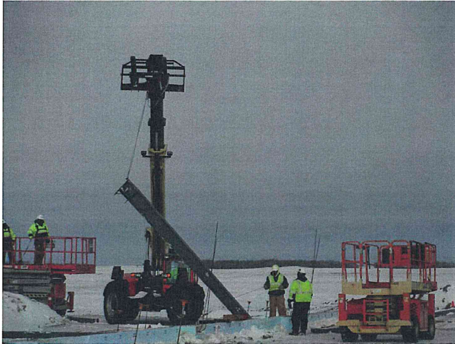
Steel Erection beginning at O&M Building
