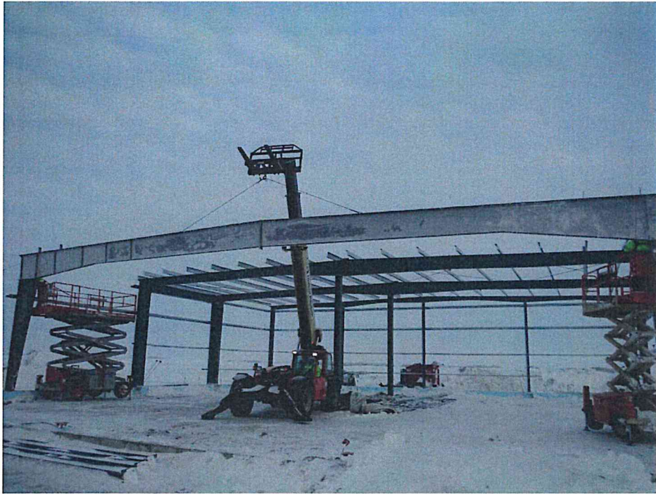
Steel Erection at O&M Building
