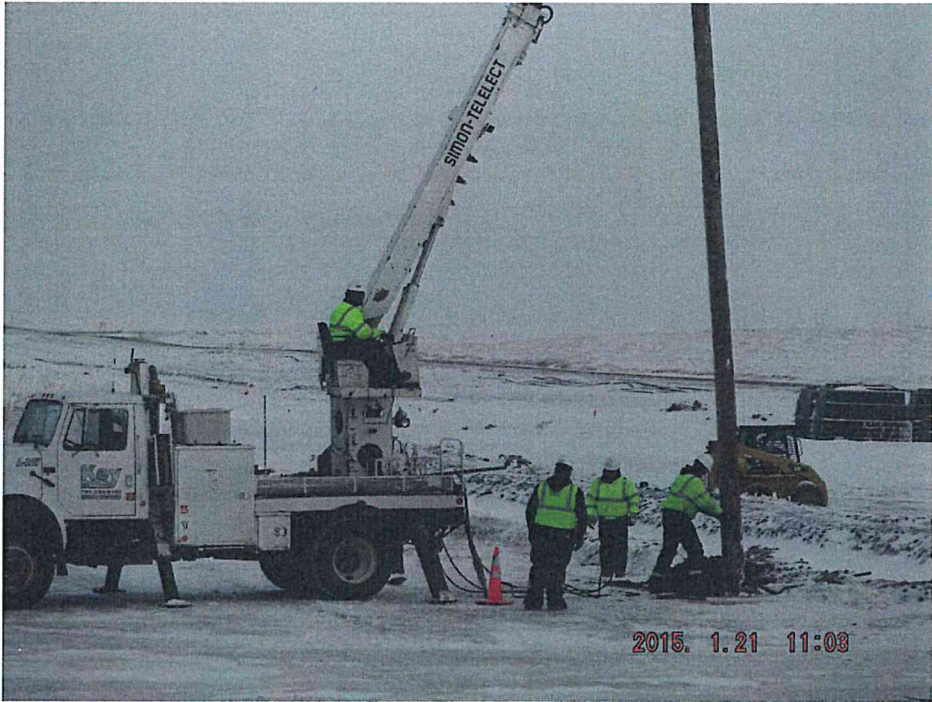
Yard lighting – pole installation
