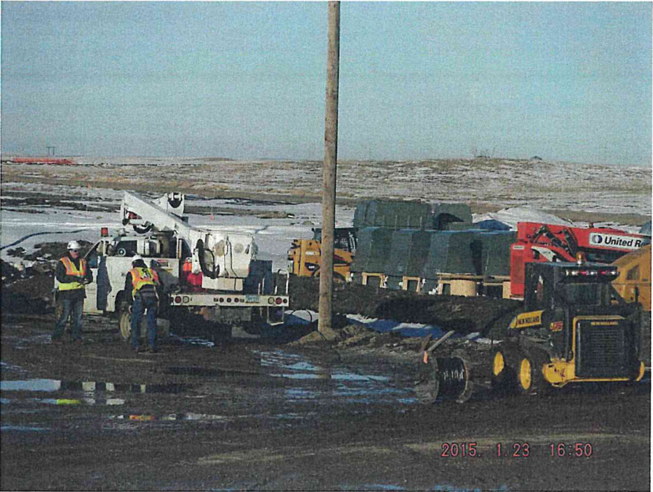
Yard lighting – Installation
