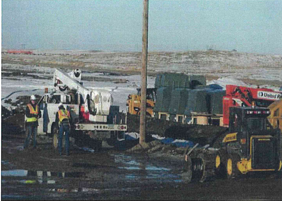
Laydown Yard Lighting Installation
