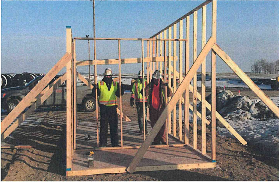
Restroom Shelter Build
