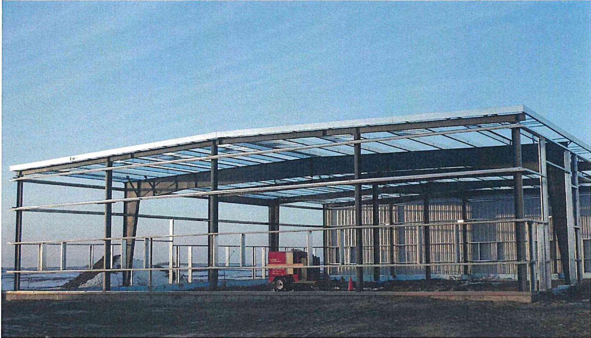
O&M Building Wall Sheeting
