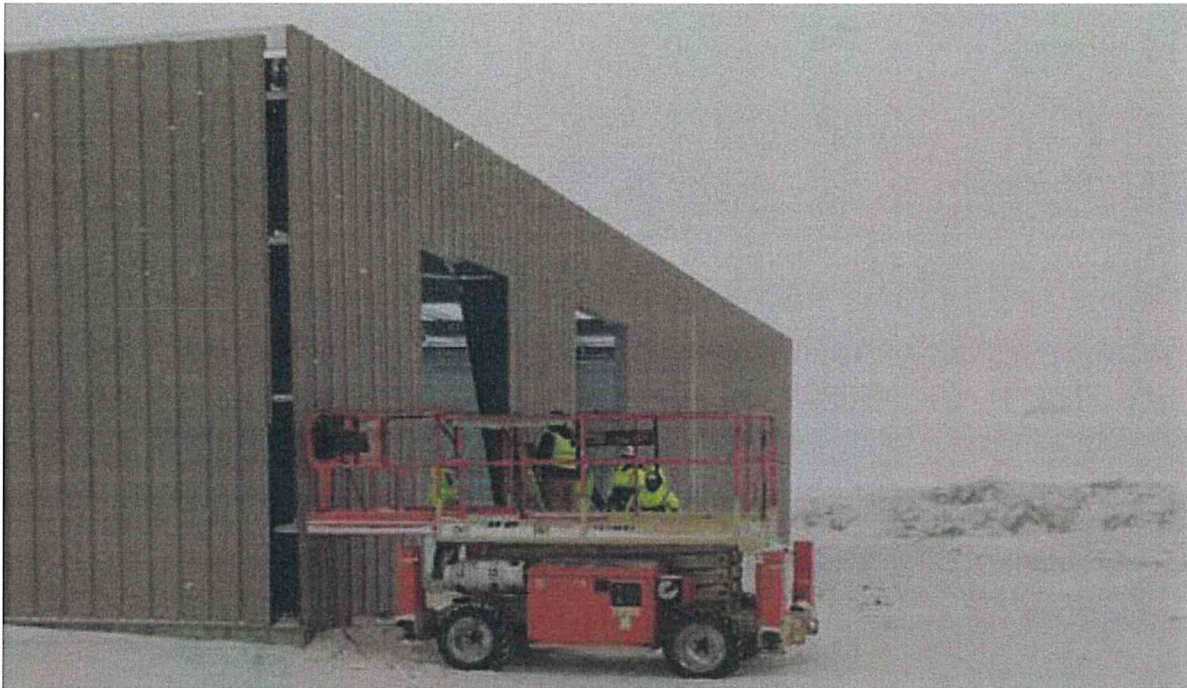
O&M Building West Wall Sheeting
