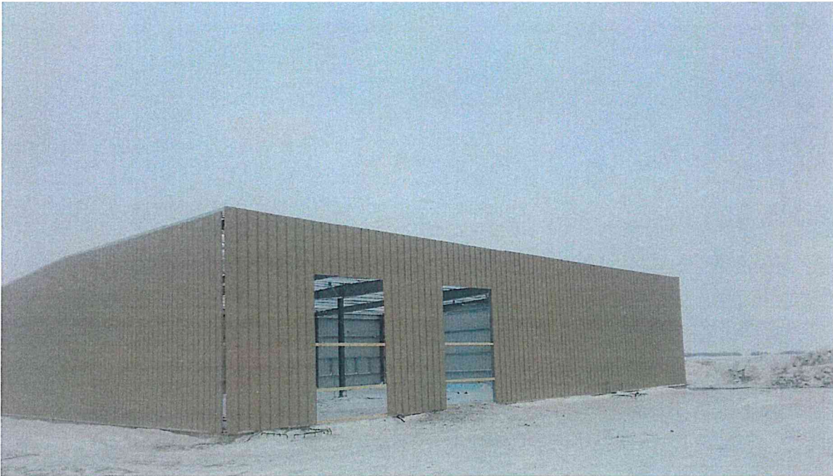
O&M Building Corner Enclosures
