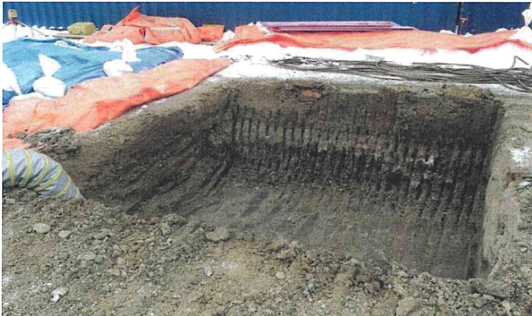
Substation – Foundation excavation
