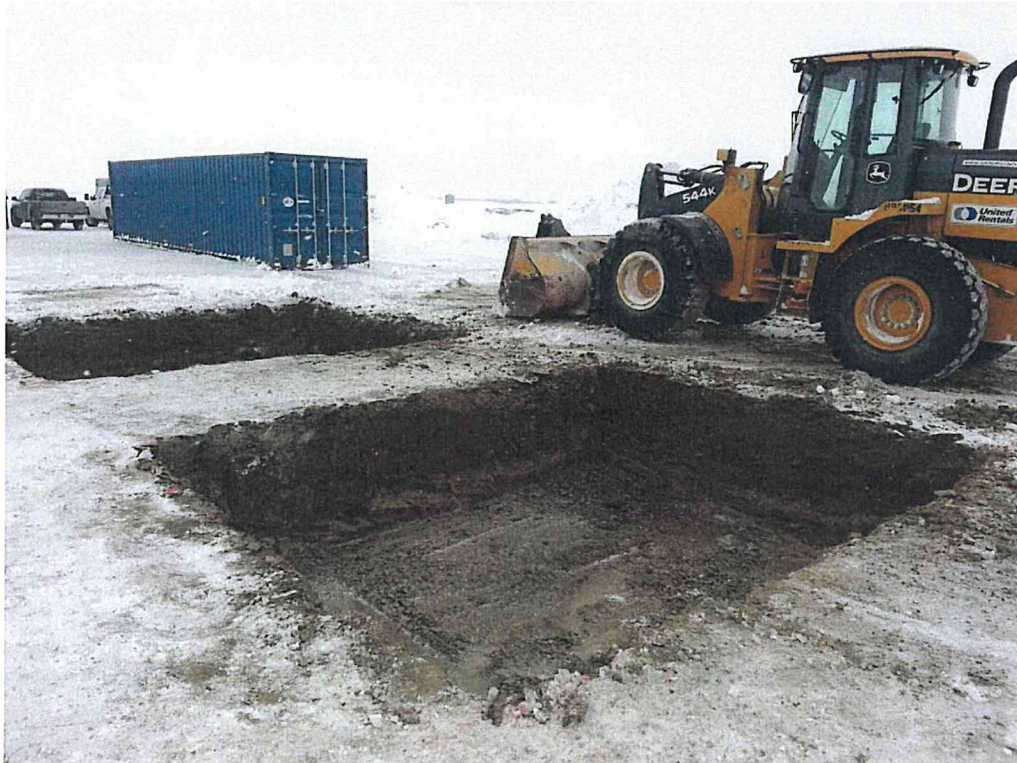
Substation Foundation excavation
