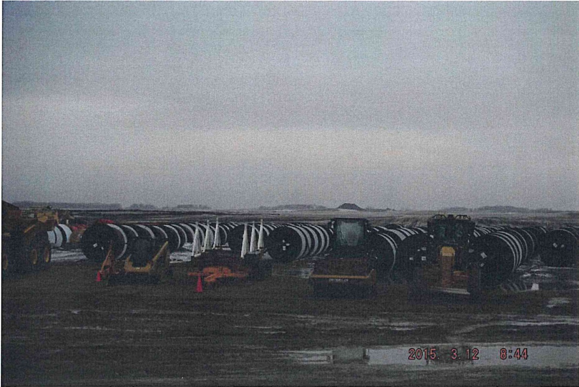
Equipment Mobilized to site
