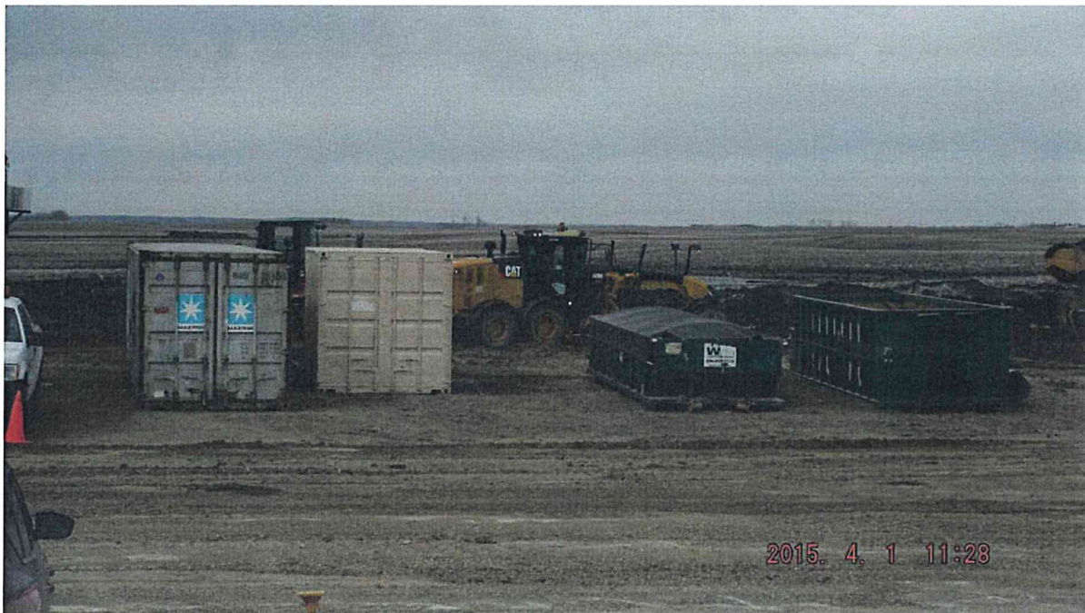
Preparing Area for Tool Trailer and Fuel Tanks – Laydown yard
