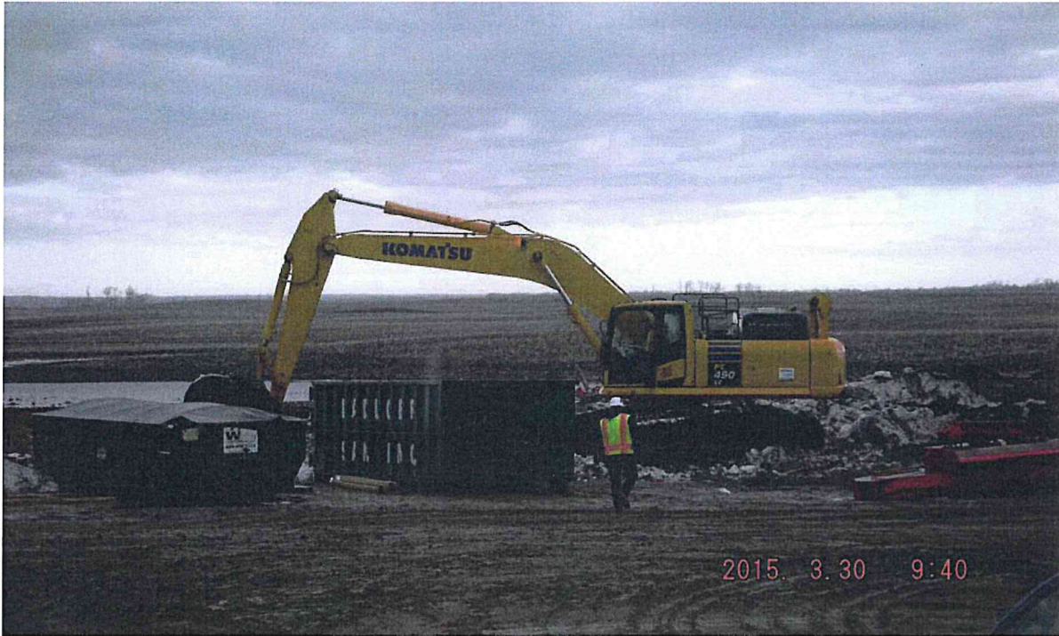
Preparing Area for Tool Trailer and Fuel Tanks – Laydown yard
