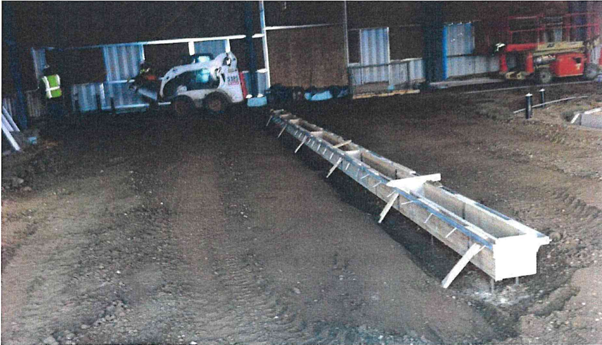
O&M Building –Shop drain formwork
