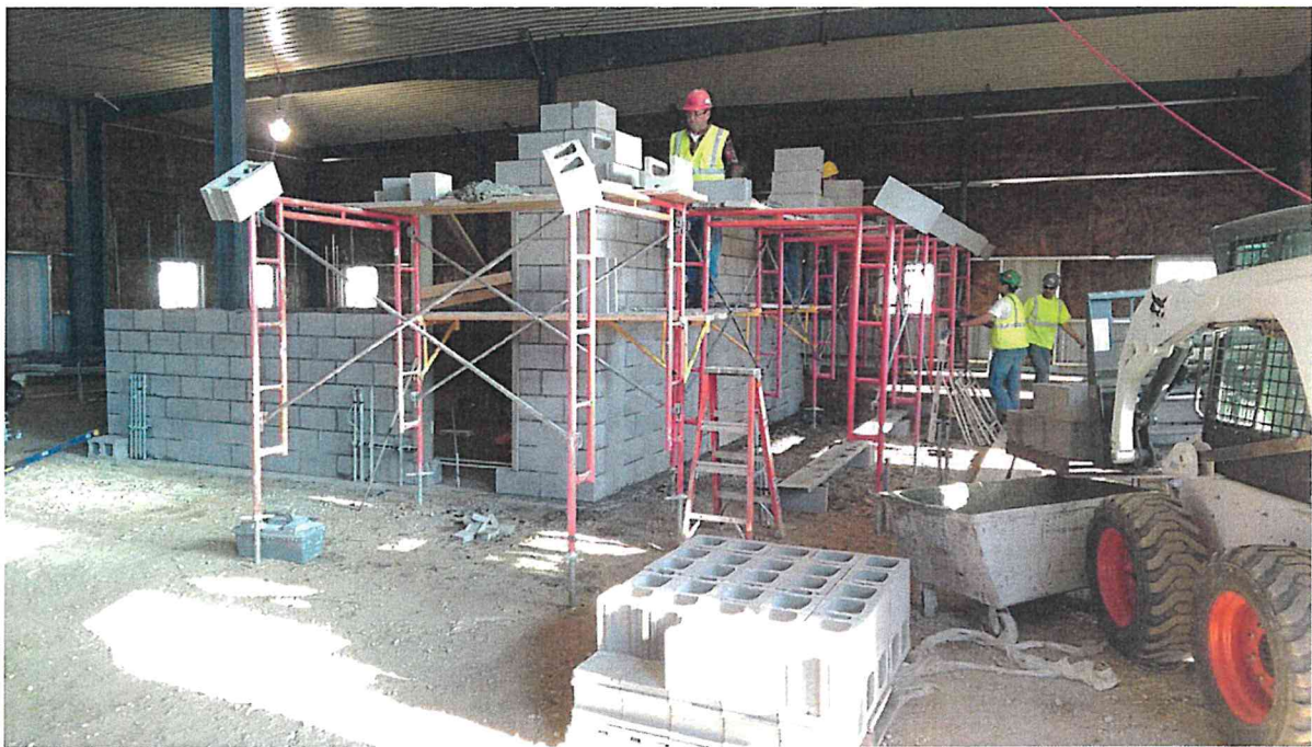
O&M Building – Storm Shelter construction
