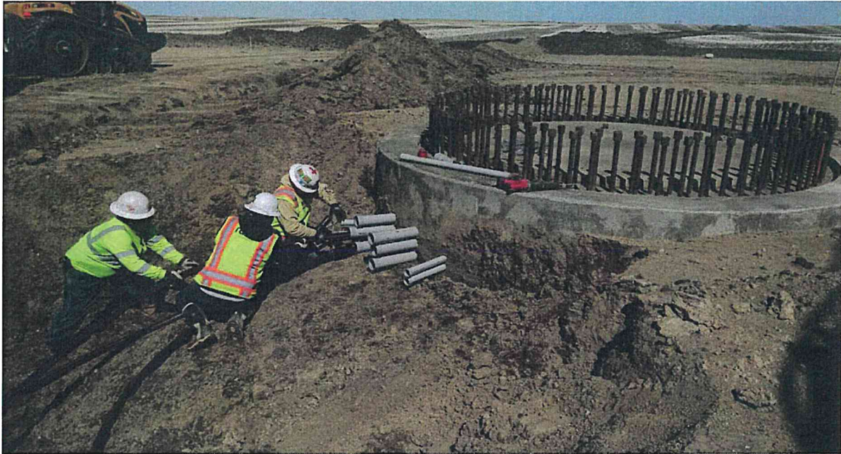
Collection System – Trenching at T26
