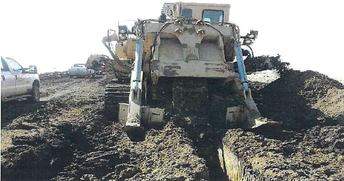
Collection System – Trenching at T26
