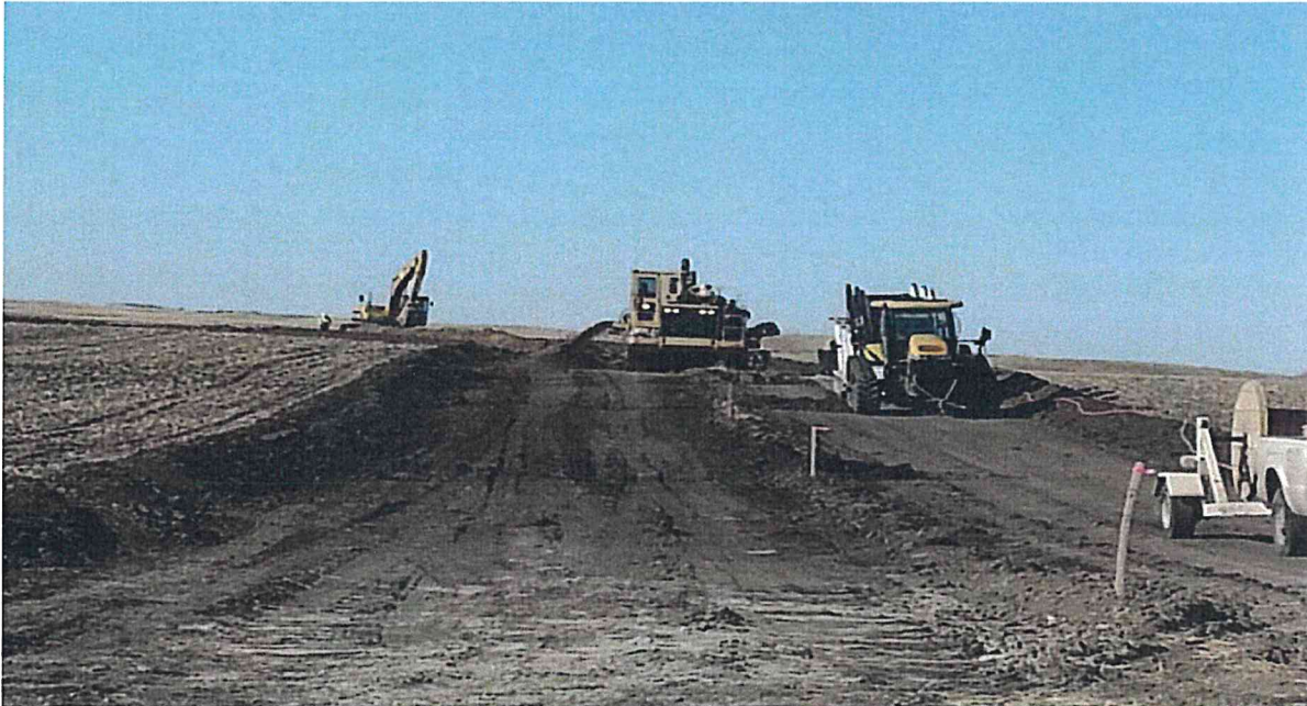
Collection System – Trenching at T24
