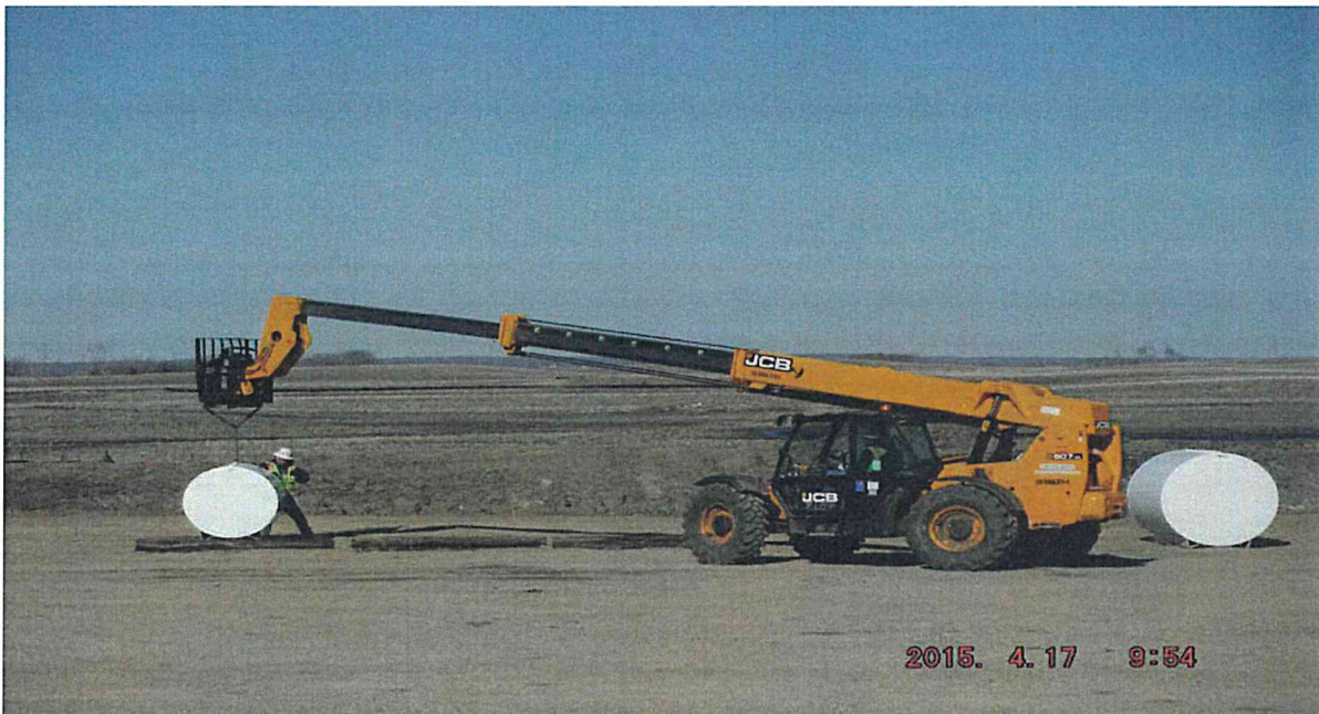
Laydown yard –Setting up fuel tanks
