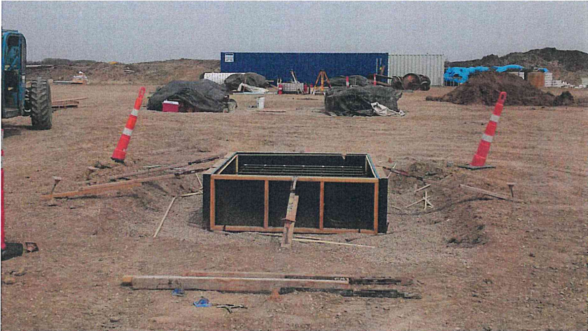
Substation - Foundation work
