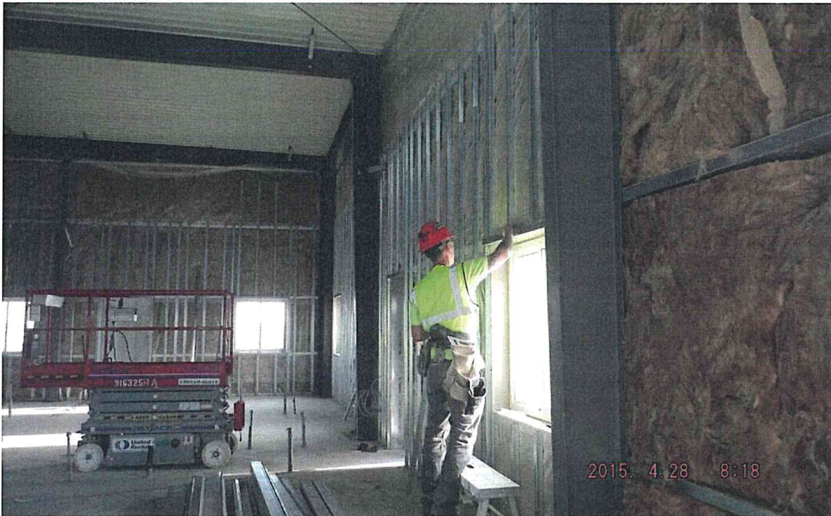
O&M Building – Window Installation
