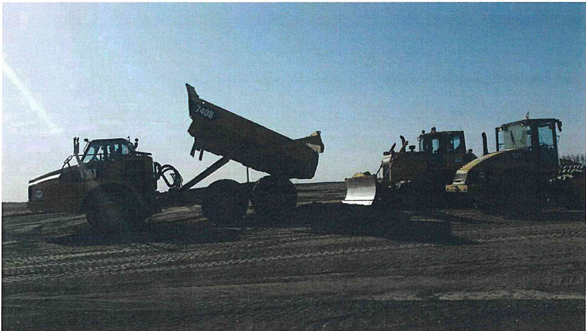
Crane pad subgrade preparation
