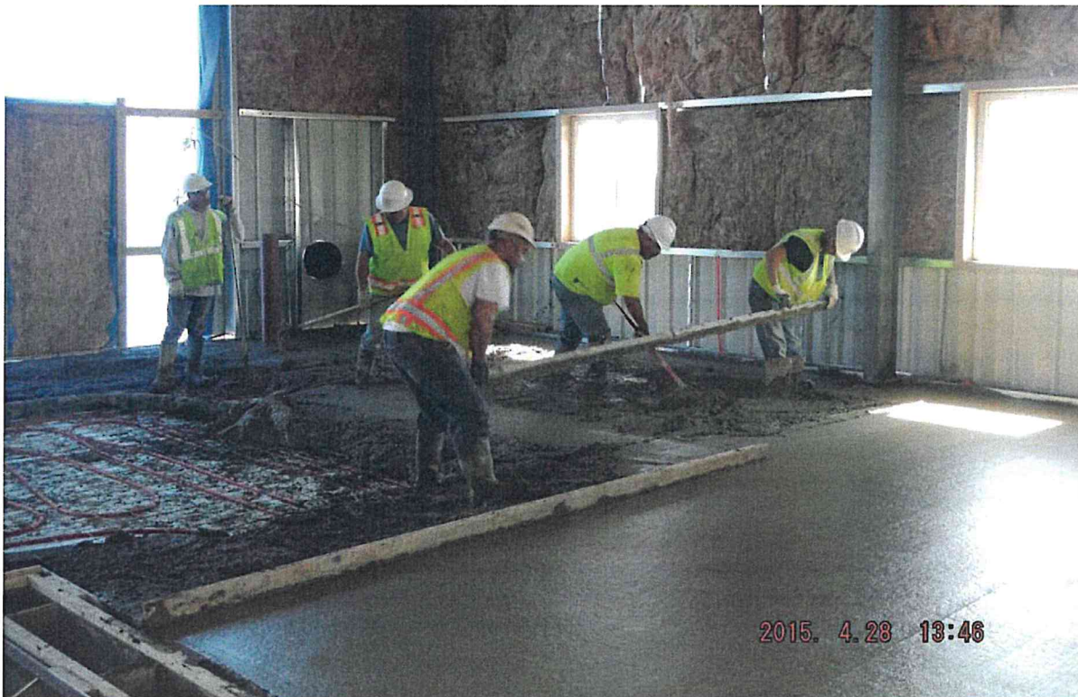
O&M Building – Floor being poured and finished.
