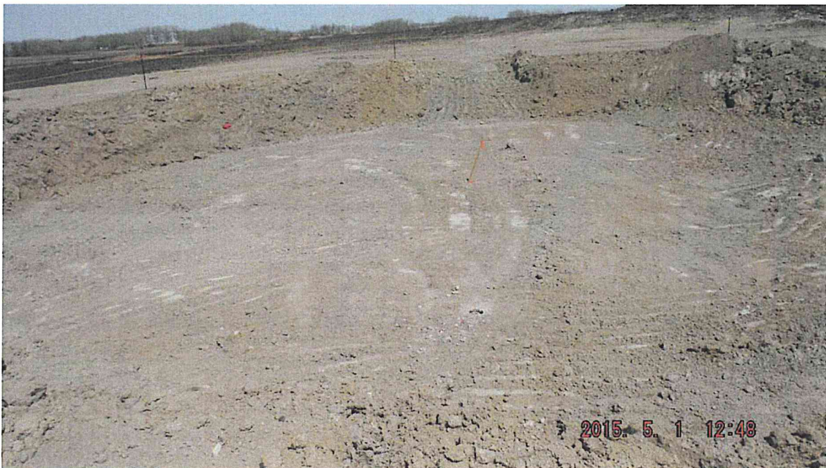
Excavation at T34
