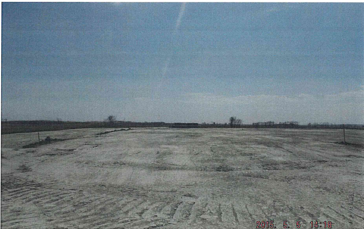
Crane pad – Subgrade at T3
