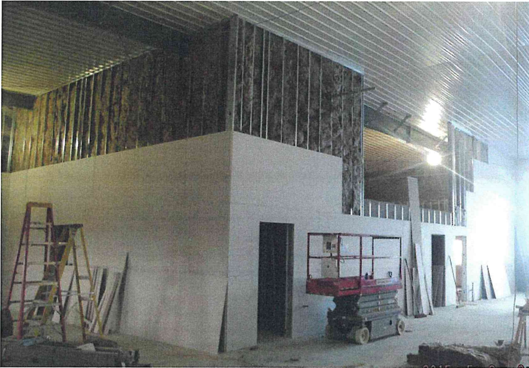
O&M Building – Sheet rock/insulation work
