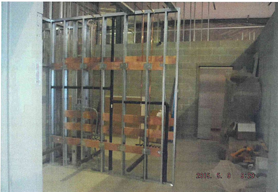
O&M Building – Storm shelter work
