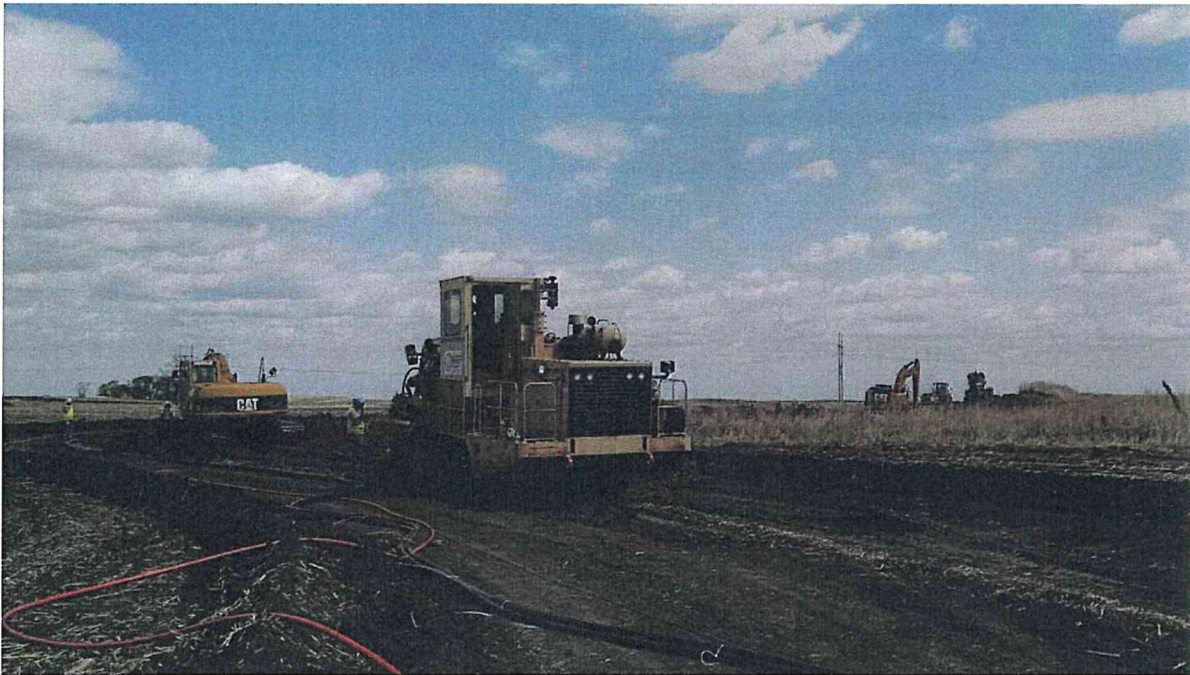
Collection System – Trenching Circuit 6
