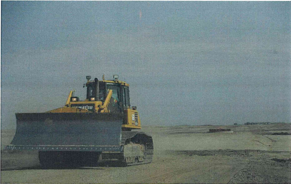
Crane pad – Subgrade preparation at T25
