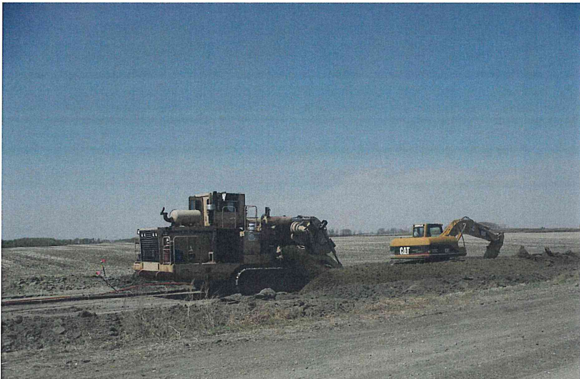
Collection System – Trenching Circuit 6
