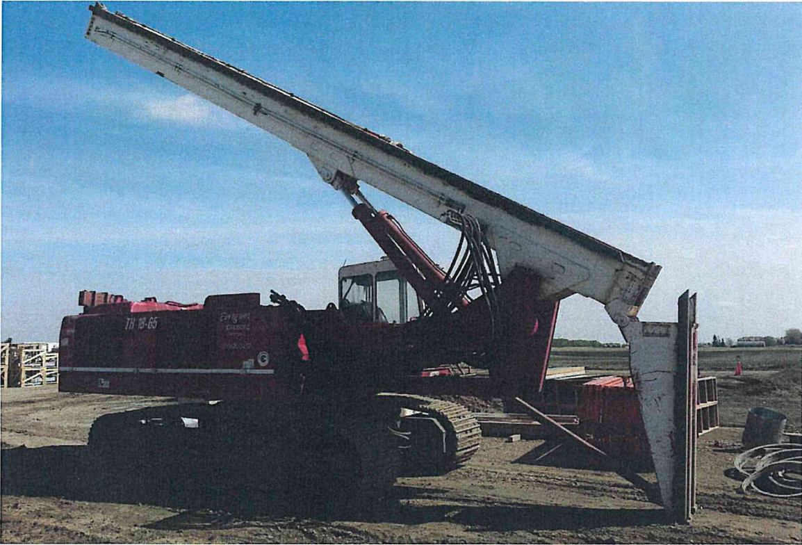
Substation – Drill rig
