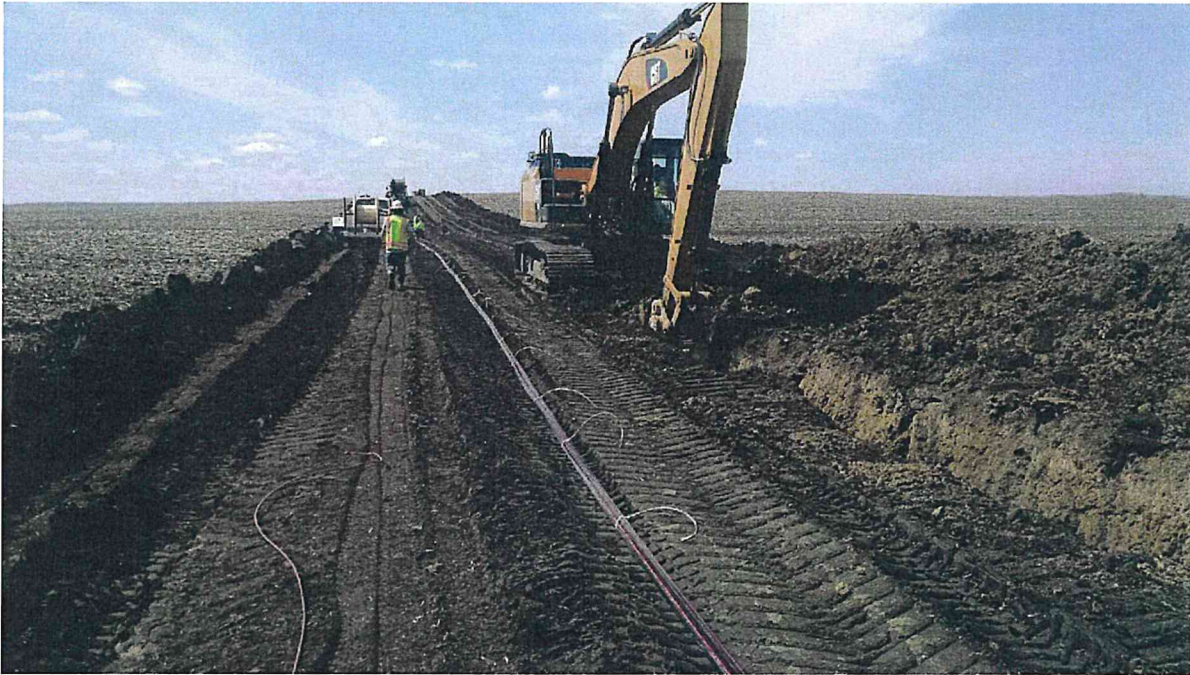
Collection System – Trenching Circuit 1A
