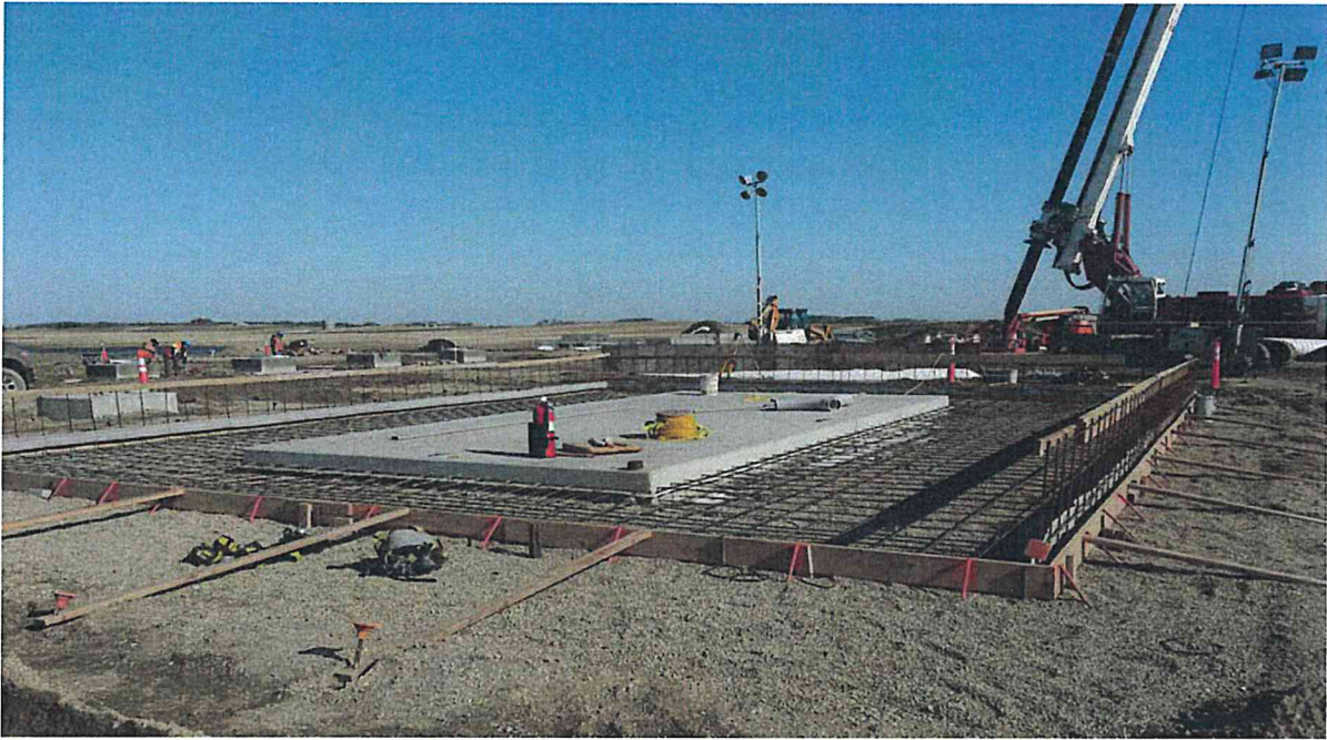
Substation – MPT Foundation
