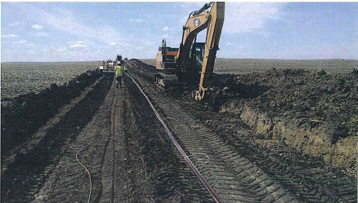
Collection System – Trenching
