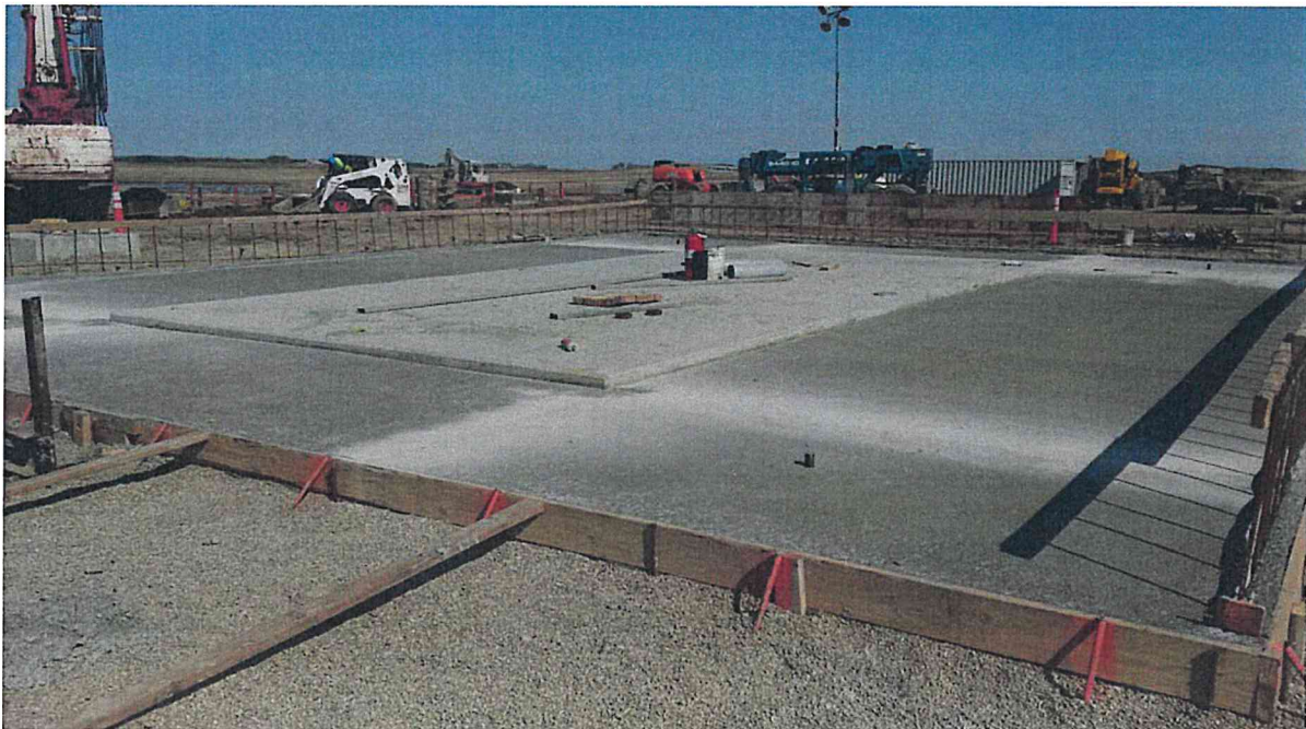
Substation – MPT foundation
