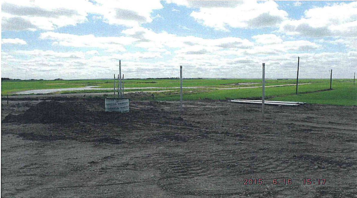
O&M Building – Fence
