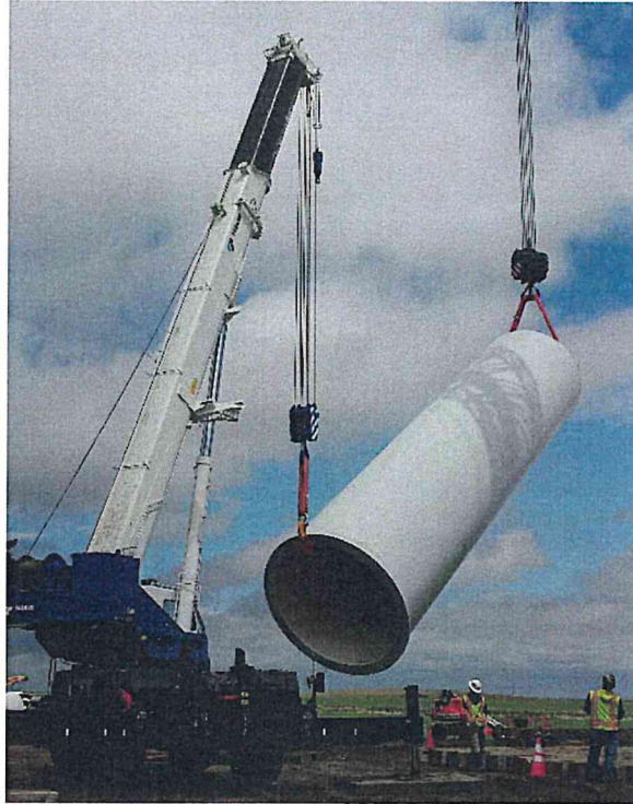
Base installation T47
