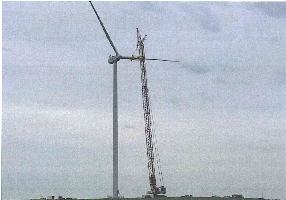
Turbine installation – T23
