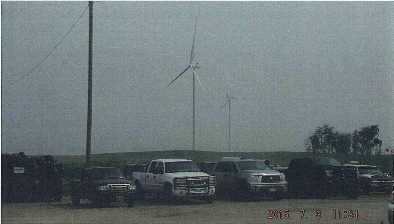
Turbines installed at T47 and T46
