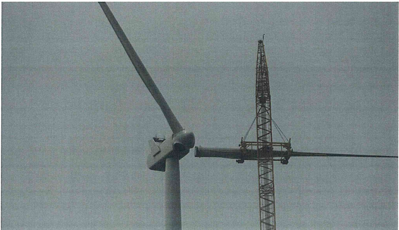
Blade installation at T45
