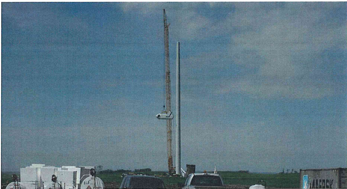
Nacelle installation at T44
