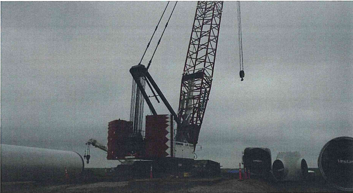
Crane and offloaded sections at T51
