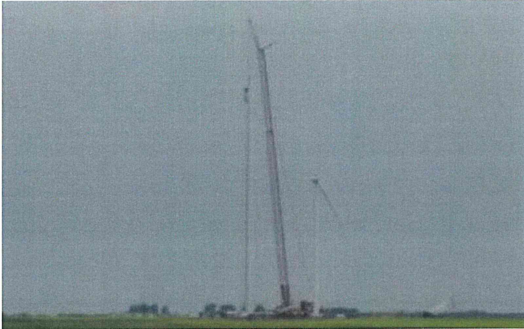
Turbine erection at T2
