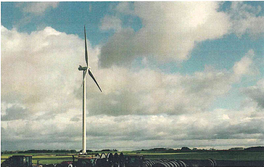
Turbine at T45
