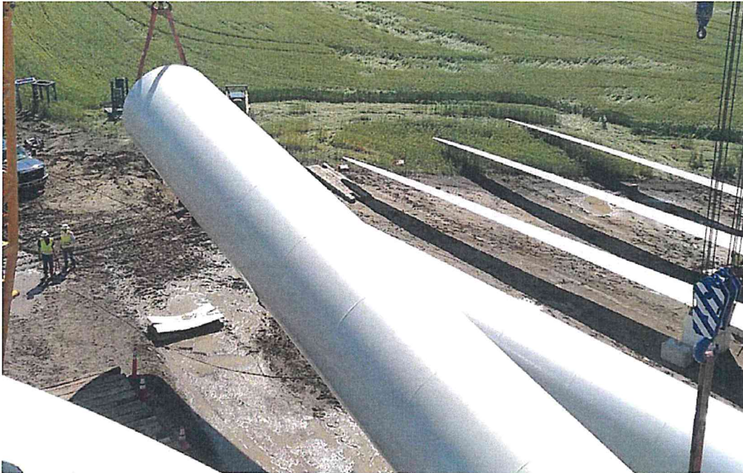
Lifting the LM at T39
