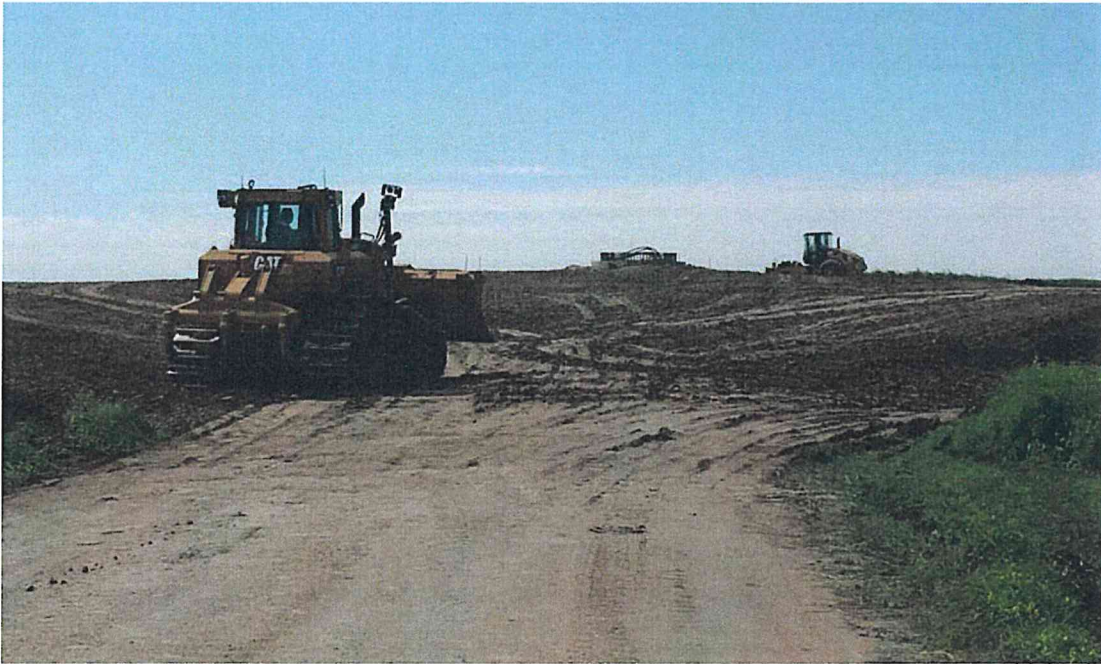
Turbine location site preparation
