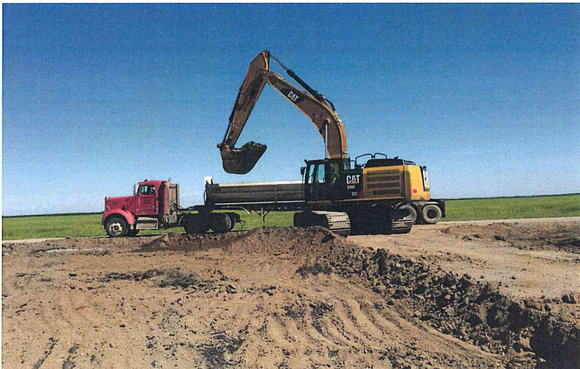
Civil Work – Removing Intersections for Reclamation
