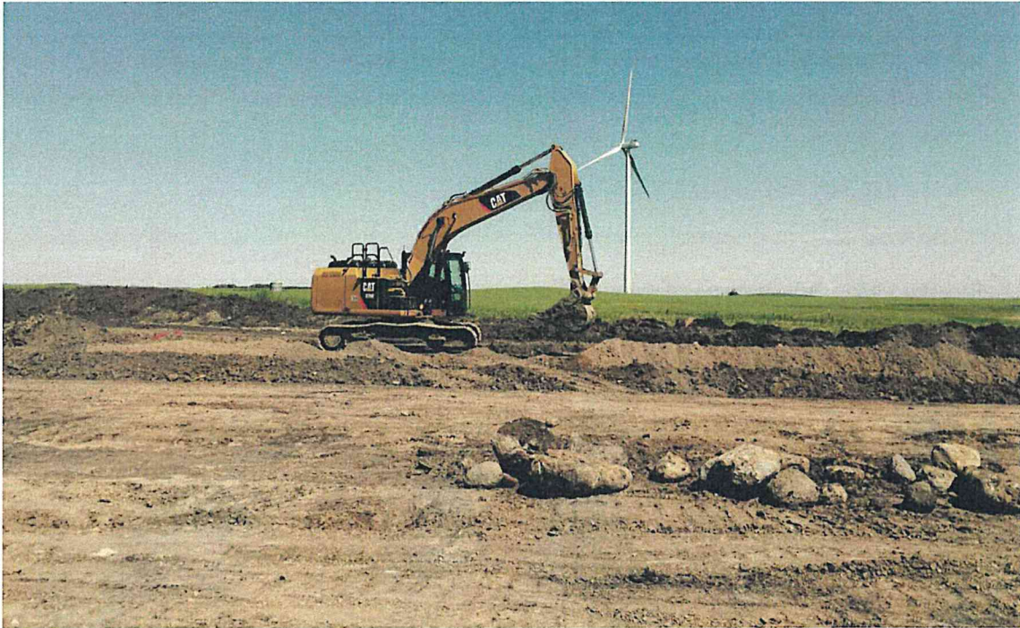
Collection – Cable trenching
