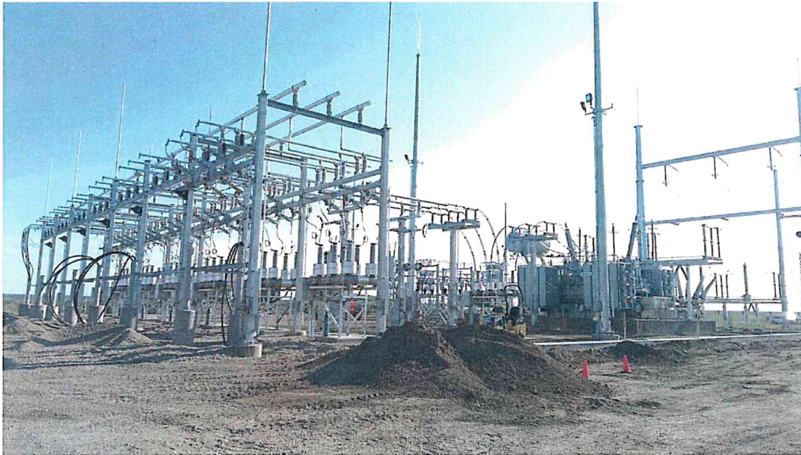
Substation – Grading work
