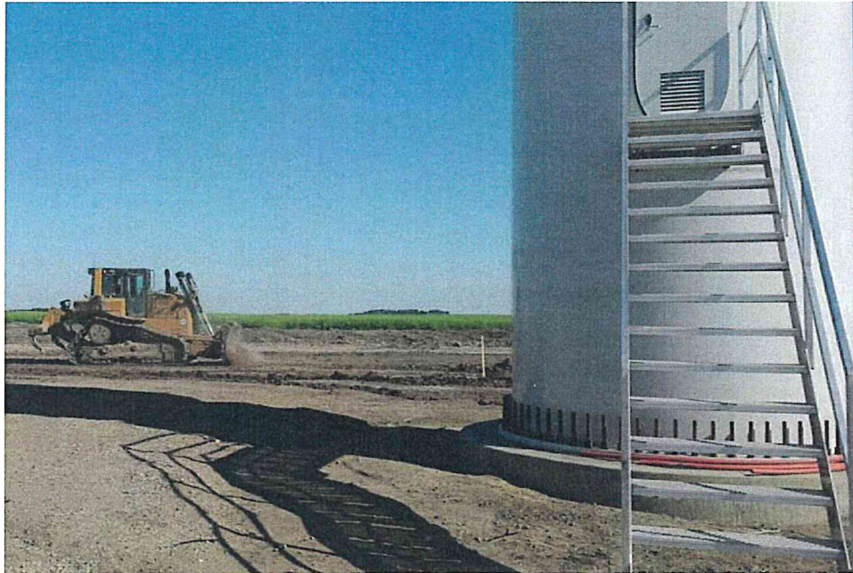
Reclamation – WTG pad
