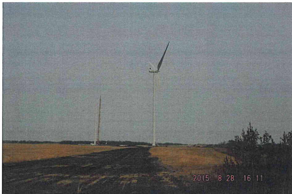
Blade installed at T10 and topping at T11
