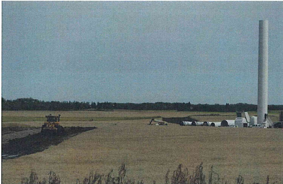
Collection line reclamation at T9
