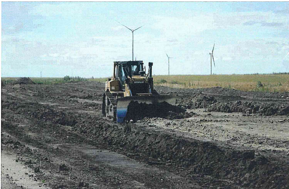
Collection line reclamation near the substation
