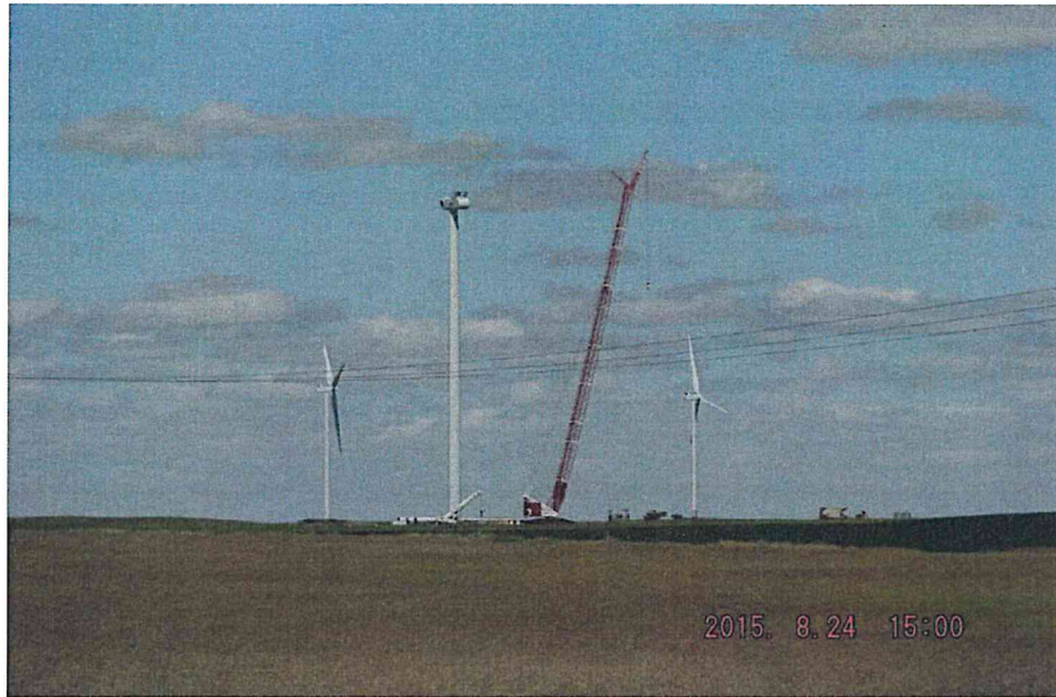
Turbine erection at T49
