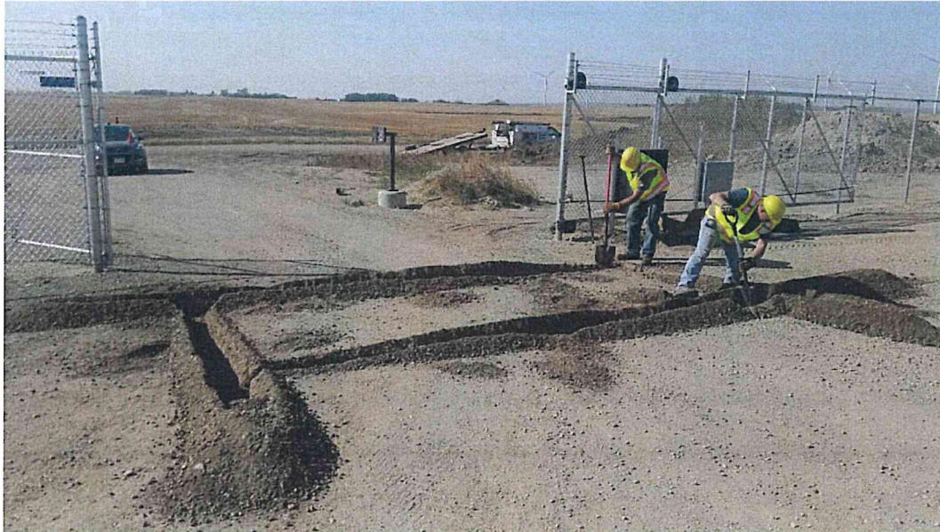
Installing the Gate Loop and the O&M Building
