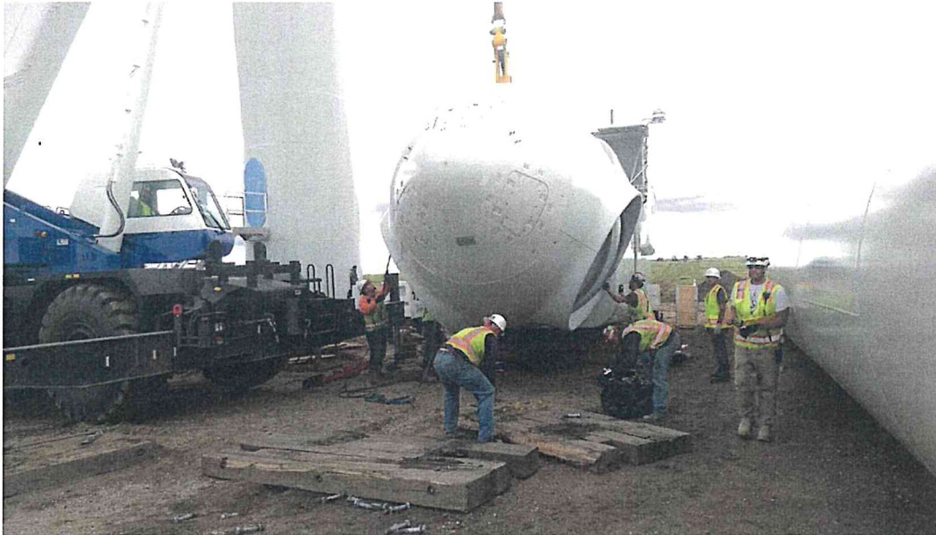
Stabbing the Hub on the Nacelle
