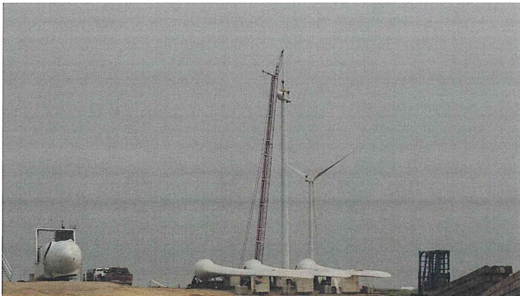
Setting the Nacelle at T67
