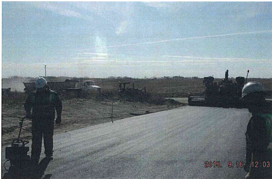
Asphalting at the O&M building
