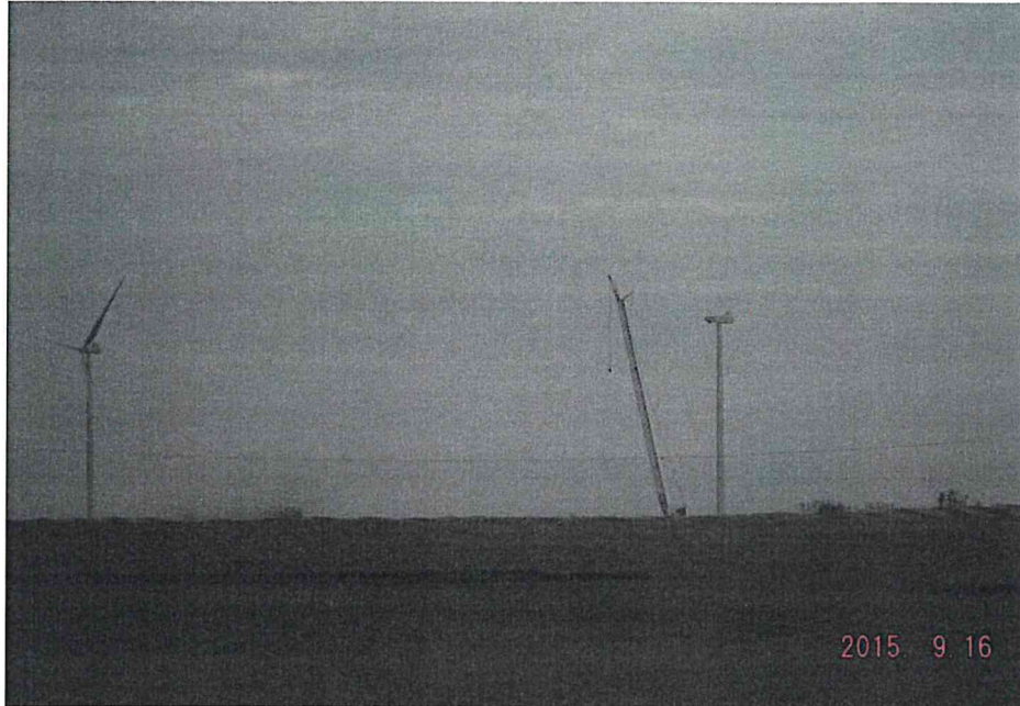
Nacelle installed at T73
