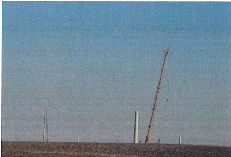
Crane 2 built at T62 & Crane 1 at T73
