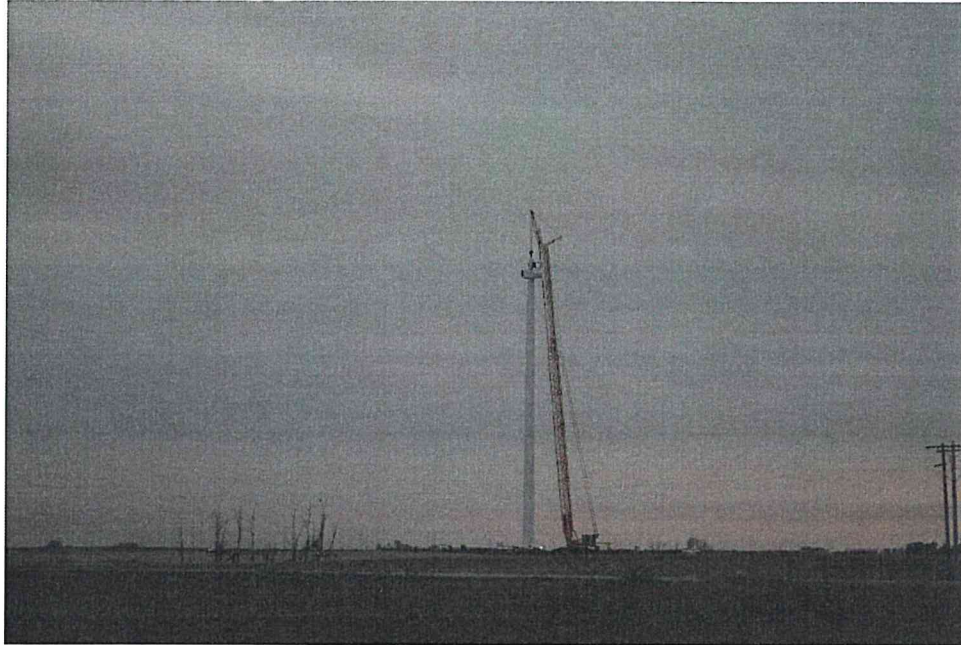
Stacking Nacelle at T61
