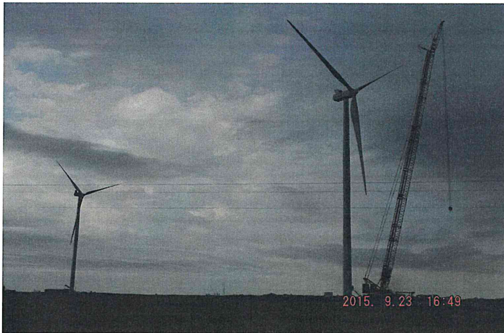
Nacelle installed at T61
