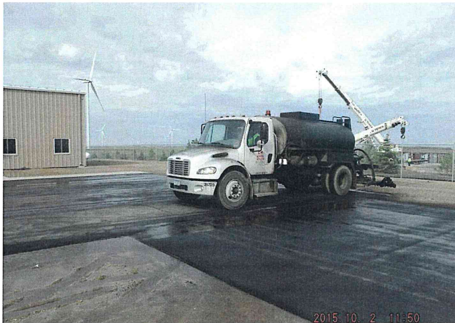
O&M Building Fog Seal
