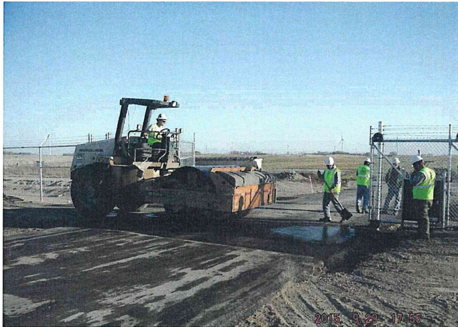
O&M Building Asphaltting
