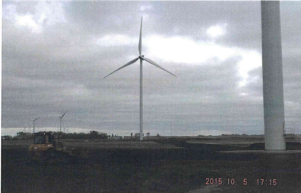
Reclamation at T16
