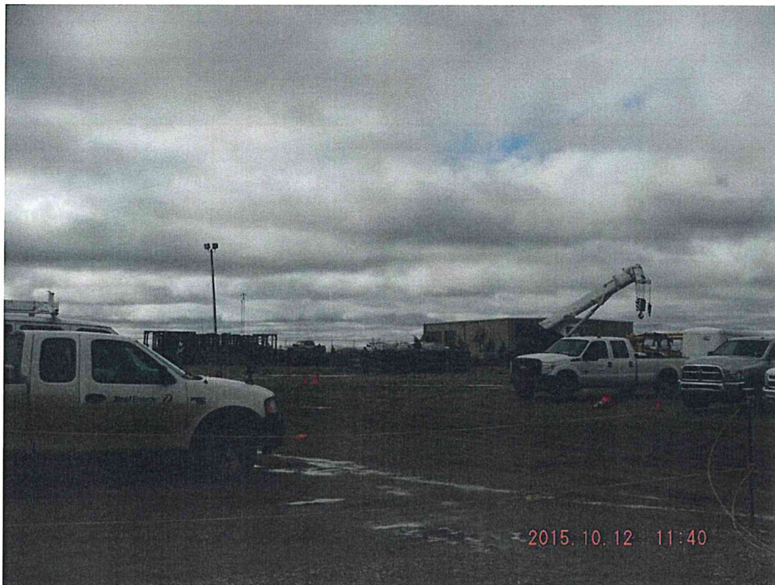
Demobilization of Turbine Yard
