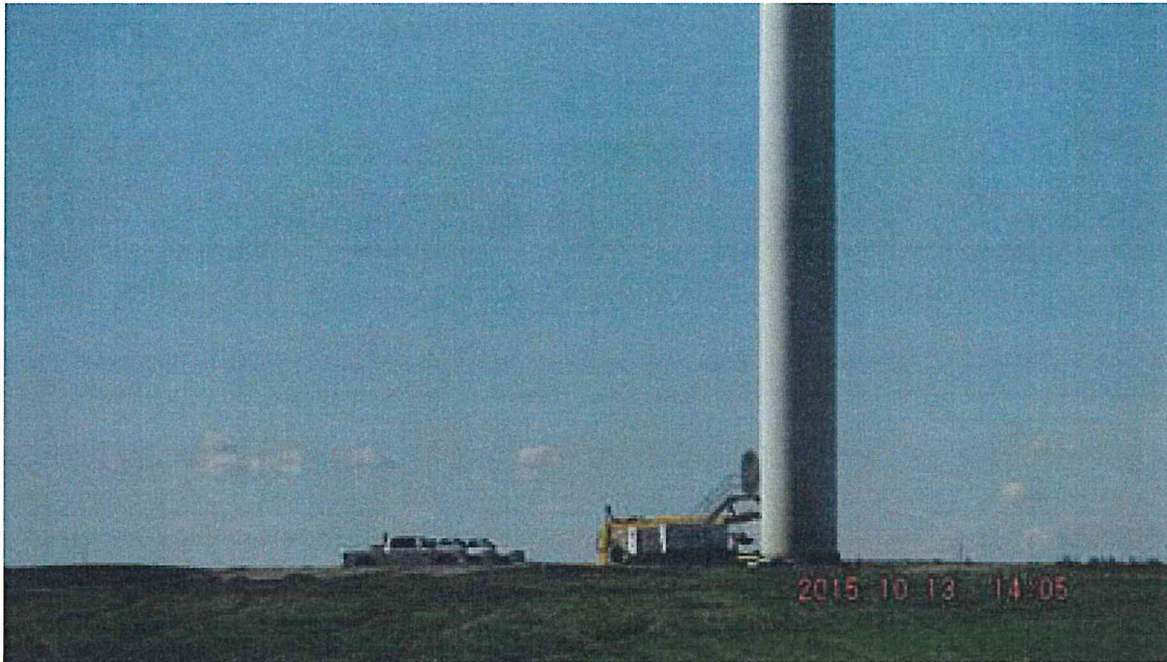
Arc Flash Testing T80
