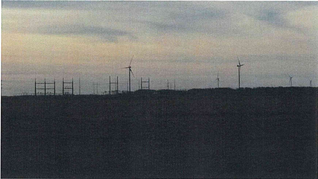
Site View of Substation
