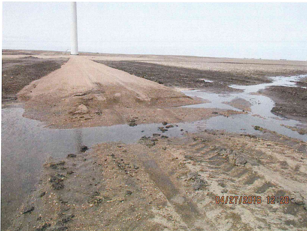
Figure 4. One of the low water crossings that was left in a cut across the road to promote runoff to follow its natural flow.
