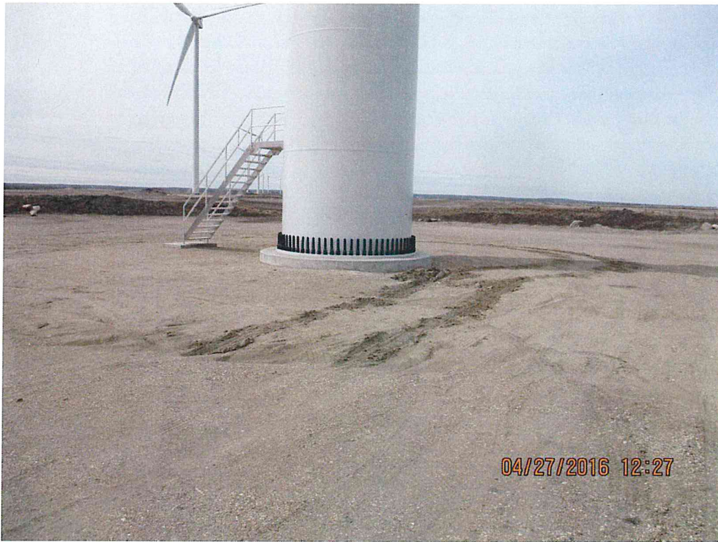
Figure 5. Clay and compaction tests still needed at T10.
