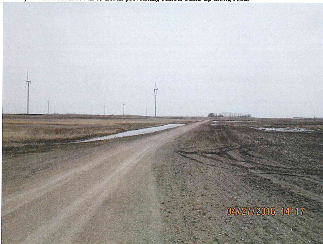
Figure 10. T26 looking south at access road that needs a low water crossing installed to help water move from west to east.
