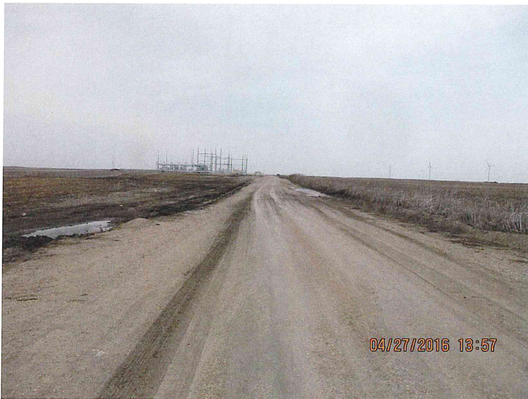
Figure 9. Looking east from the access road to the substation. Work will be done to provide adequate flow from south to north preventing runoff build up along road.
