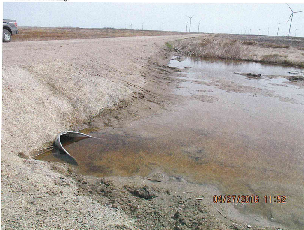
Figure 2. Photo of a turning radii that needs further reclamation. Culvert clean out, replace and add topsoil, score and seed, and lay ECB to existing vegetation.
