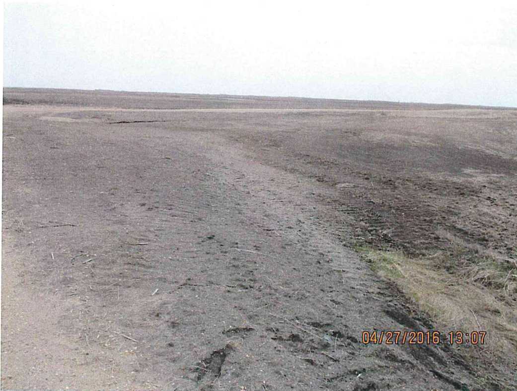
Figure 7. Turning radii that needs to be redone. Establish ditch, new black dirt, seeding, and ECB.
