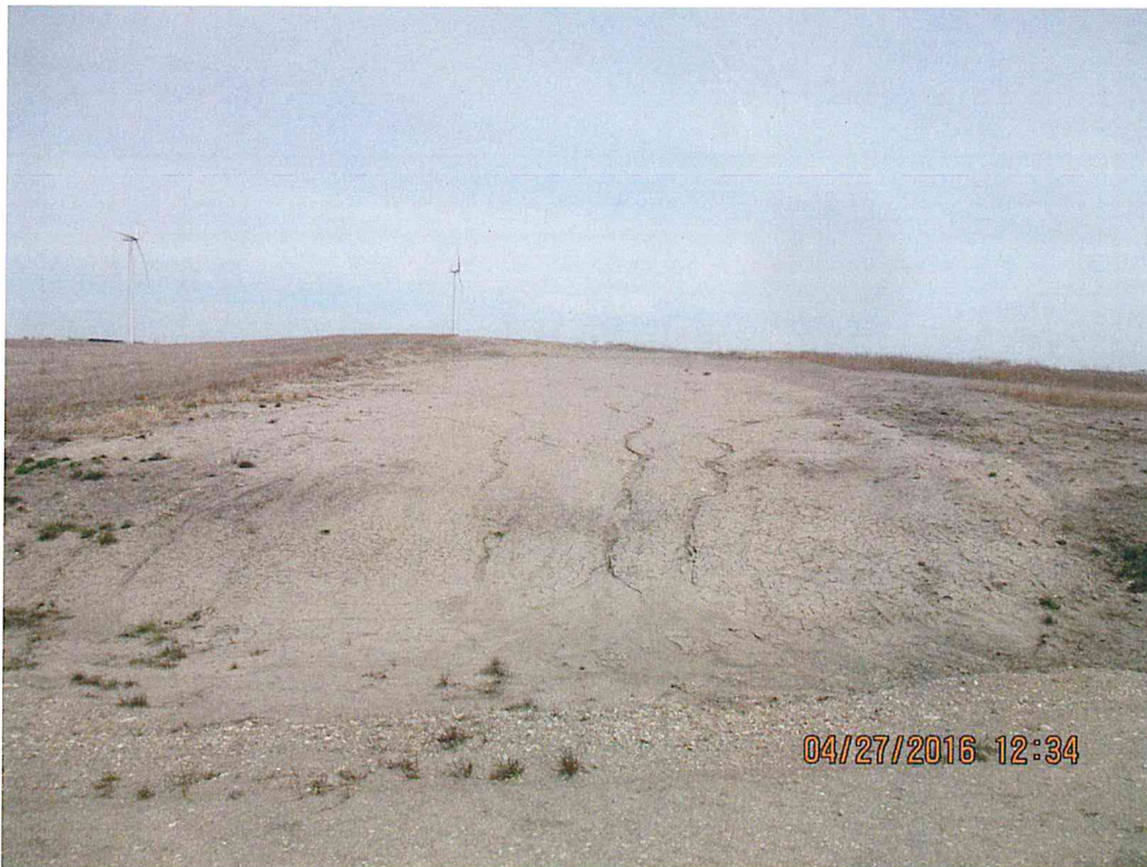
Figure 6. Crane walk area for moving across the road. Ditch will be re-established and the soil removed.
