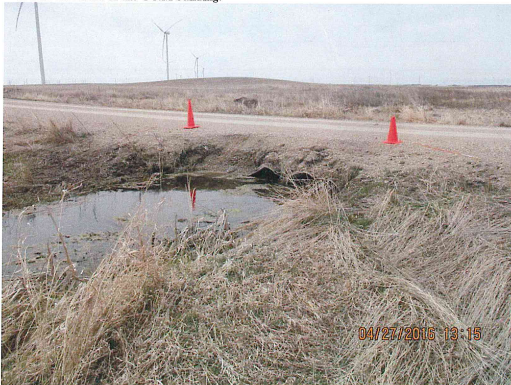
Figure 14. Culverts under 53rd Ave NE where road maintenance will be performed.
