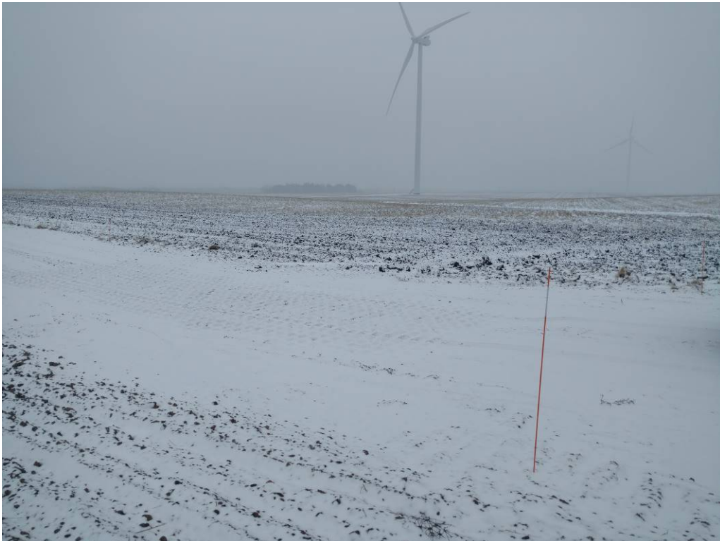
Figure 3. Photo of revetment mat at low water crossing to Turbine 19 (looking northeast).
