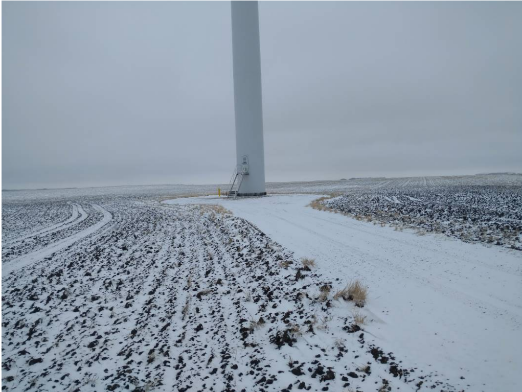
Figure 8. Typical turbine pad. Photo taken facing north at Turbine 25. Turbine pad has been reduced from construction and surrounding area graded to match existing contours.
