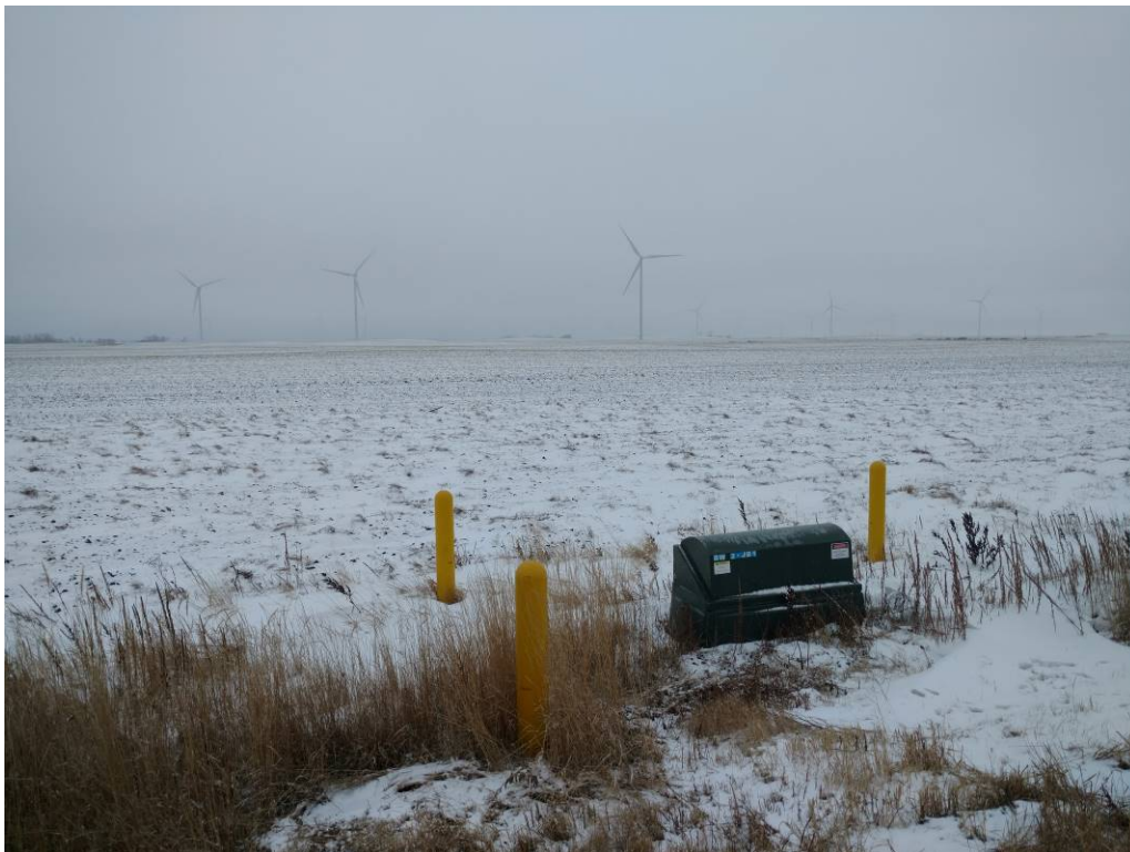
Figure 9. Photo taken facing west from Kyle Road, looking along collection line. Line route has been restored and matches surrounding contours.
