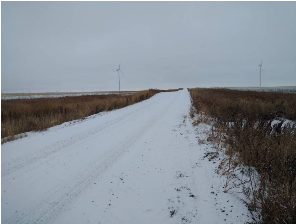
Figure 13. Photo taken facing north at same location as Figure 12. Road has been restored after construction.
