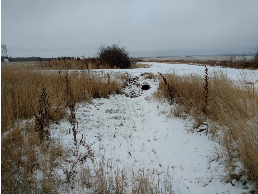
Figure 6. Photo taken facing south at intersection of 47 th Ave NE and access road to Turbine 15. Road ditch has been reclaimed and riprap placed at mouth of culvert.
