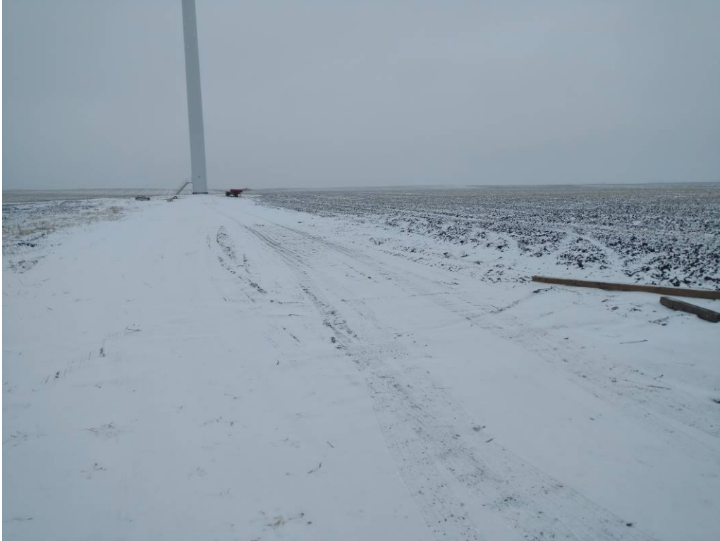
Figure 4. Photo taken looking west towards Turbine 6. This location was noted in the May Construction Inspection report (Figure 4) as needing fixing. A revetment mat has been placed in the low-water crossing. Construction debris is due to generator replacement that occurred a few days prior.
