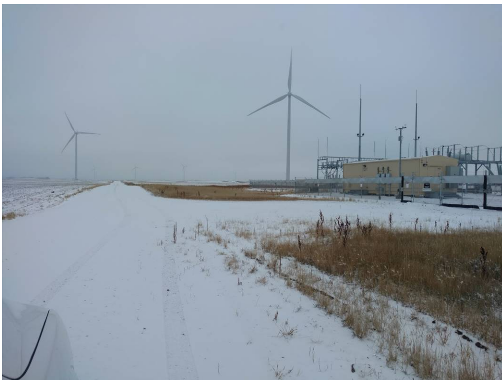
Figure 11. Photo taken facing west along access road to substation. Area surrounding substation has been revegetated.
