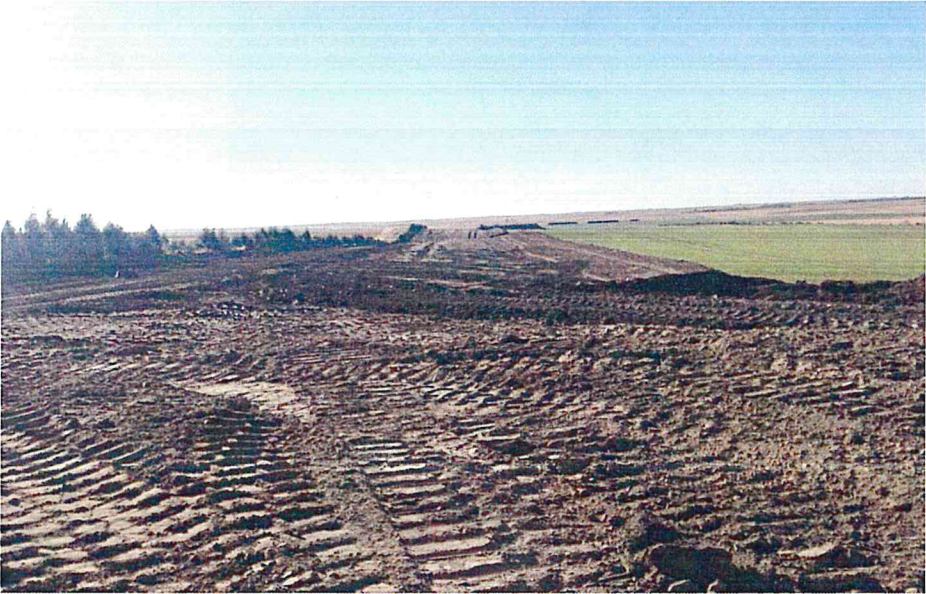
Civil- Access Road from Turbine Pad 2 to Turbine Pad 1
