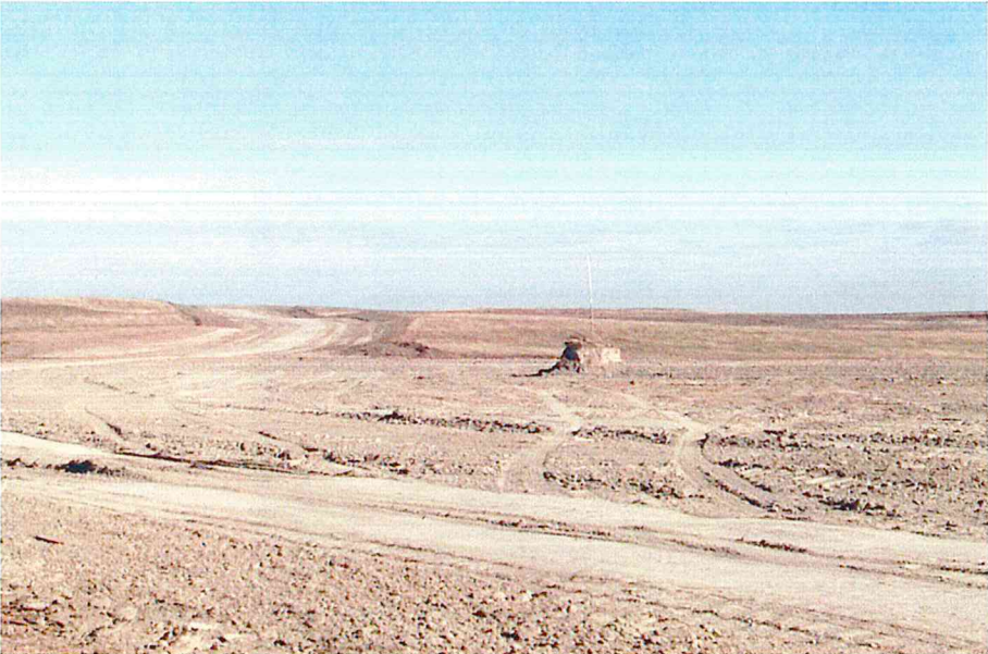
Civil- Cut/Fill Turbine Pad 4
