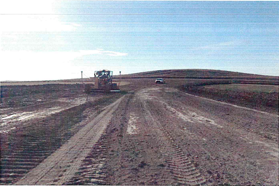
Civil- Entrance to Turbine 9 and Turbine 10 Access Road
