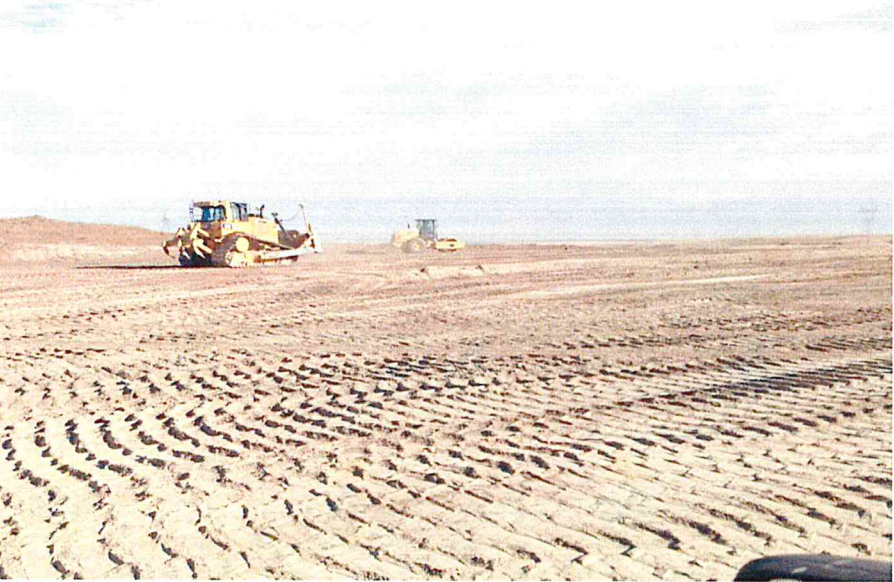
Civil- Cut/Fill Turbine Pad 10
