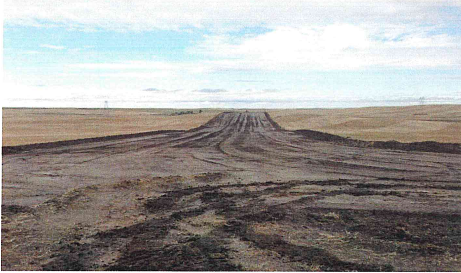
Civil- Grading Substation Access Road
