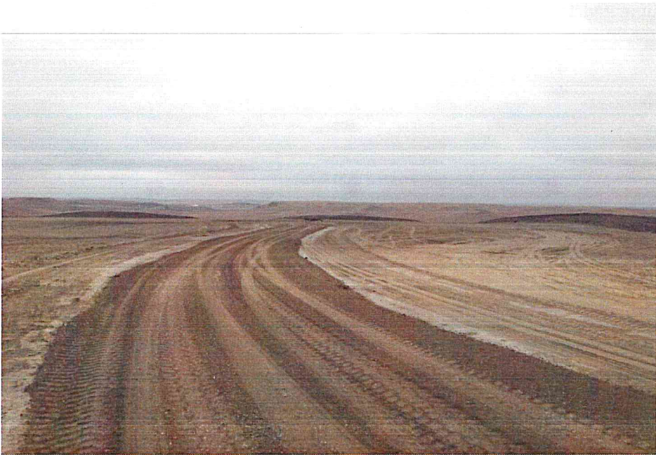
Turbine Pad 17 - Access Road Cap
