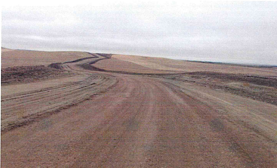
Finished Access Road between Turbine Pad 4 and 3
