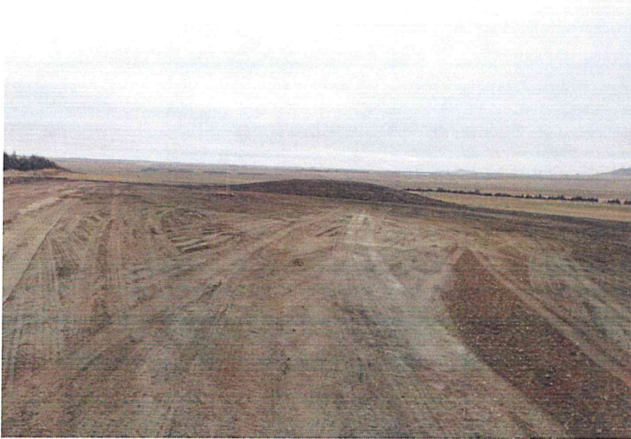
Access Road to Turbine Pad 1
