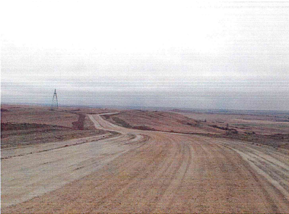
Finished Access Road to Turbine Pad 18
