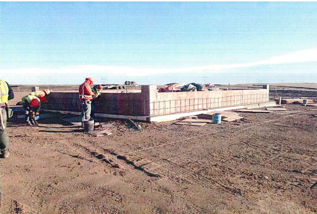
Main Power Transformer Foundation Work
