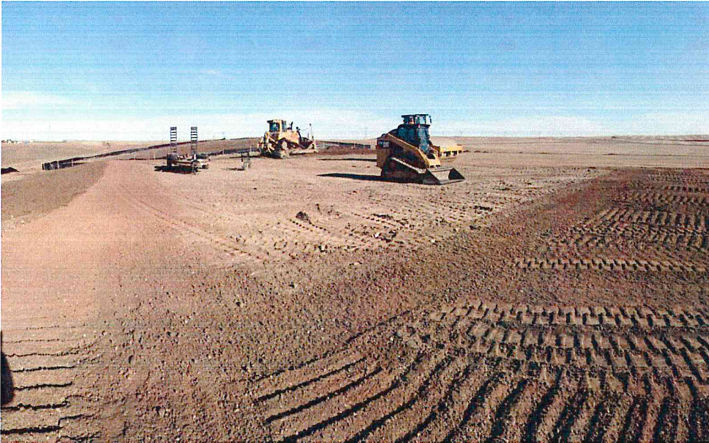
O&M Building Yard Aggregate placement
