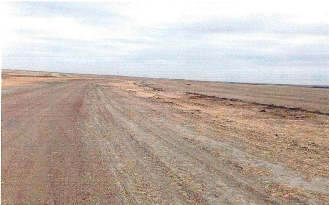
Placing and Binding Mulch between Turbine Pad 13 and 14
