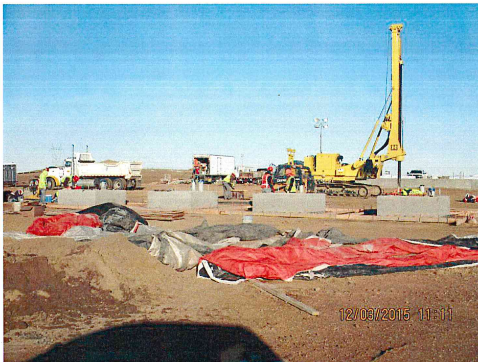
Figure 4. Construction of substation and secondary containment for grounding transformers.
