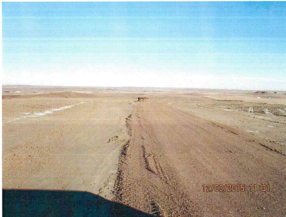
Figure 8. Photo of preliminary grading of the turbine pad at T20.
