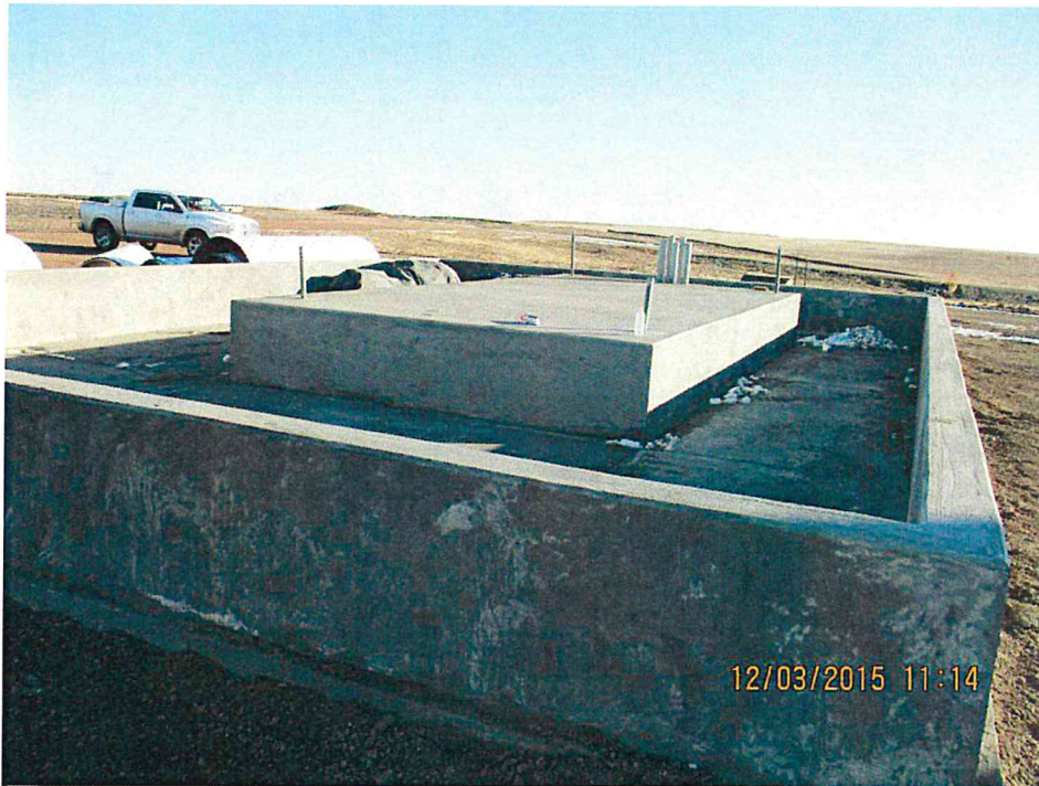
Figure 5. Construction of substation and secondary containment of the step up transformer.
