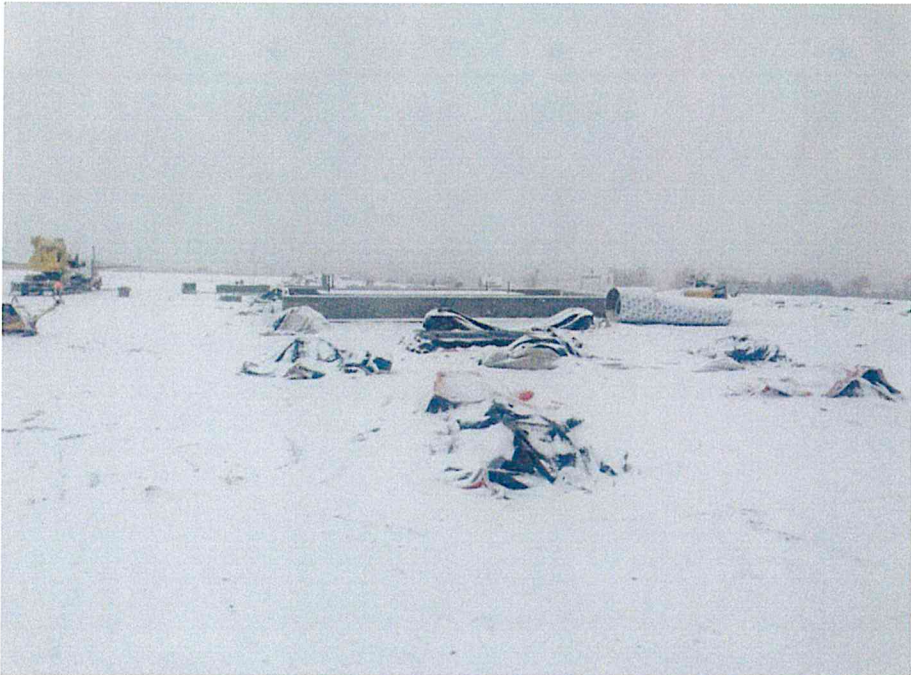
Pier Foundation wrapped in blankets for curing.
