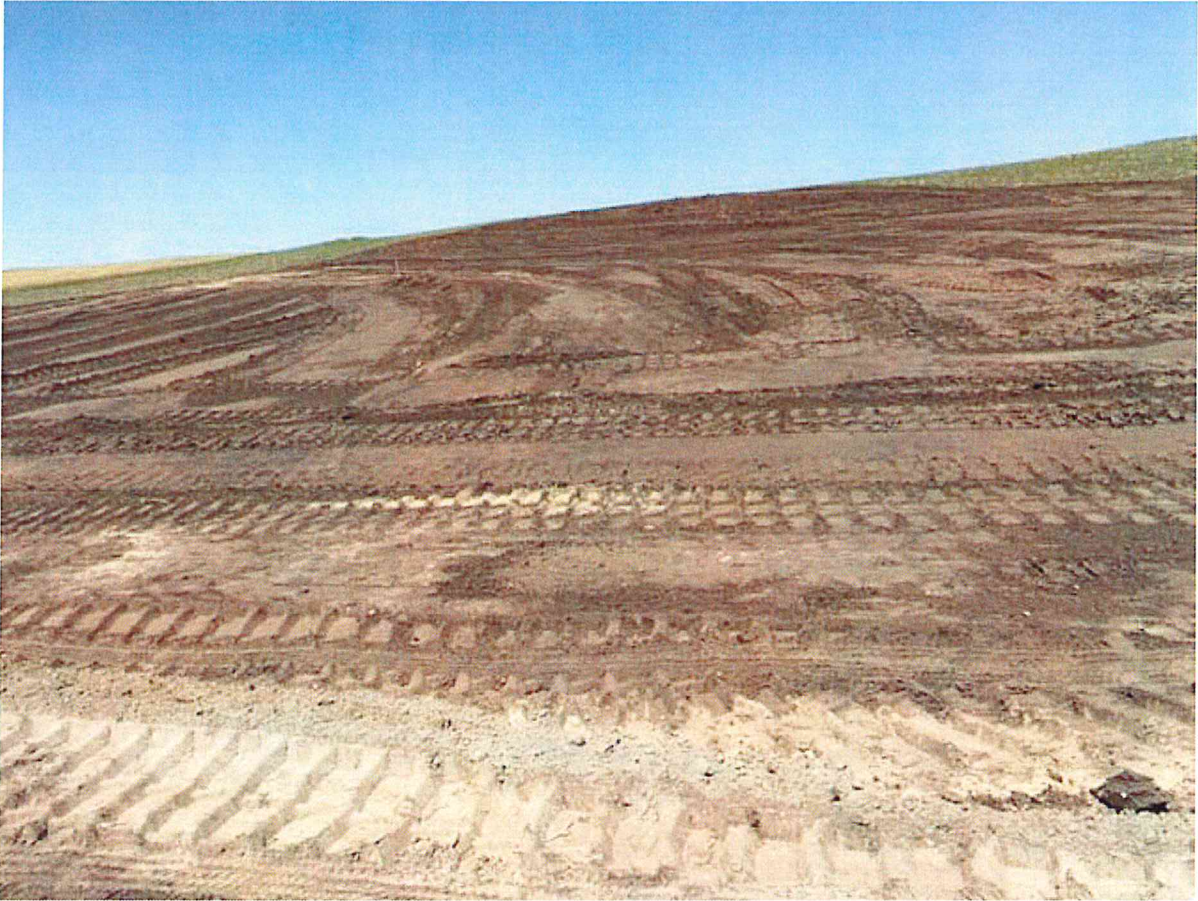
Pad site stripping
