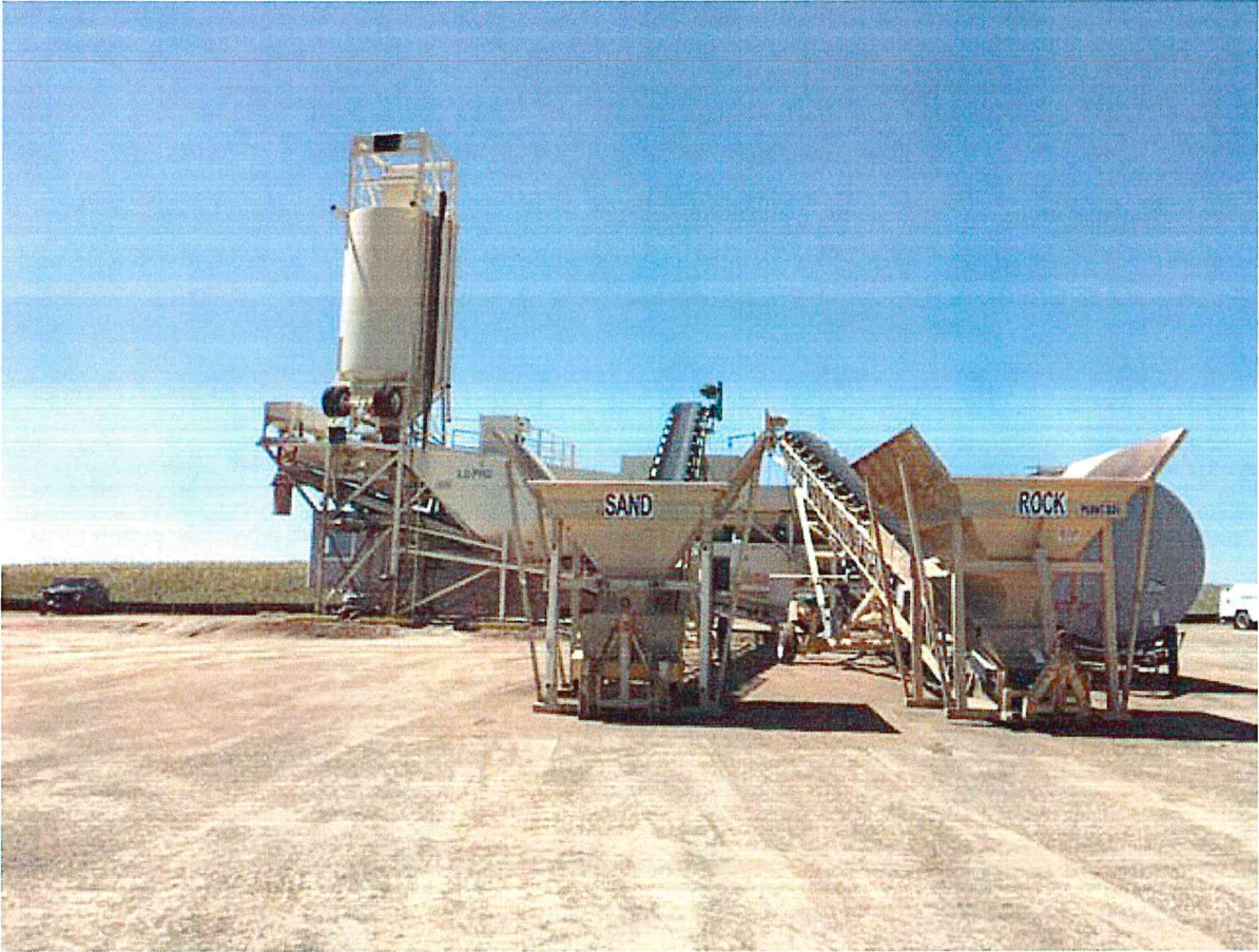
Mobile batch plant set-up
