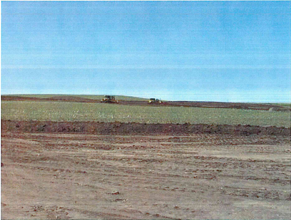
Access road cut/fill
