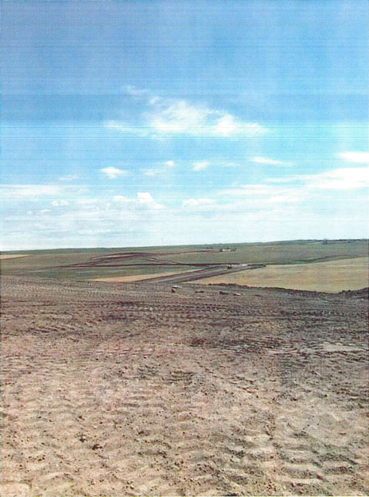
Pad Site Topsoil Stripping and Grading
