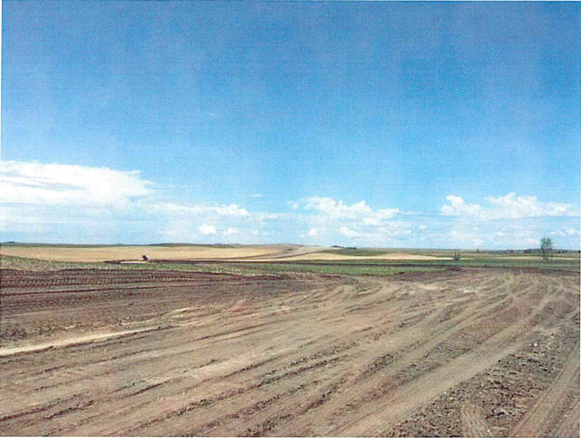
Access Road Topsoil Stripping and Grading
