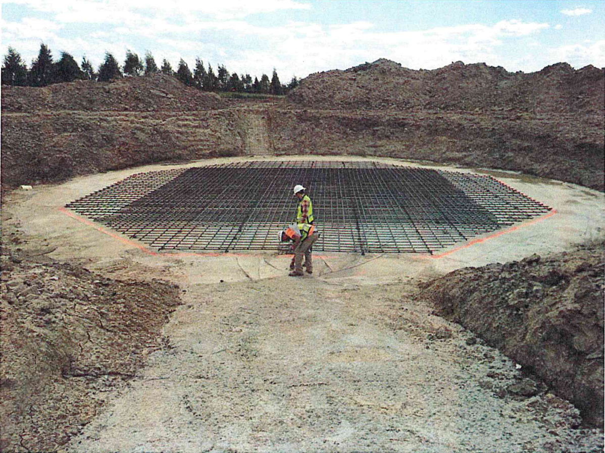
Foundation 1 Mud Mat and Bottom Rebar Mat
